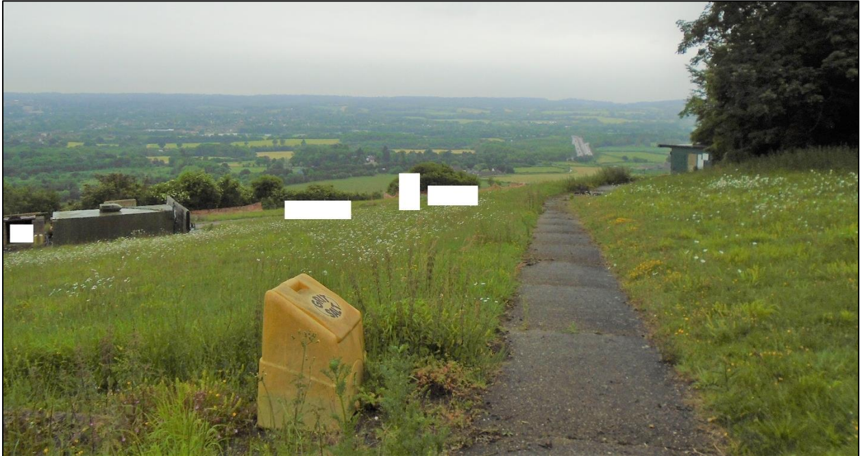
Plate 9: View towards Chevening and M25 (facing south-west) from the south-west of the fort
