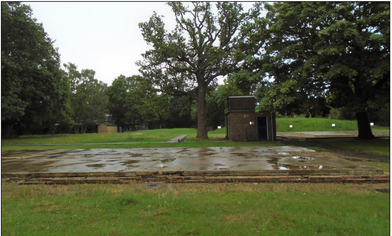
Photograph 6: View of building foundations on Crow Drive (located at c. TQ 49453 59054)
