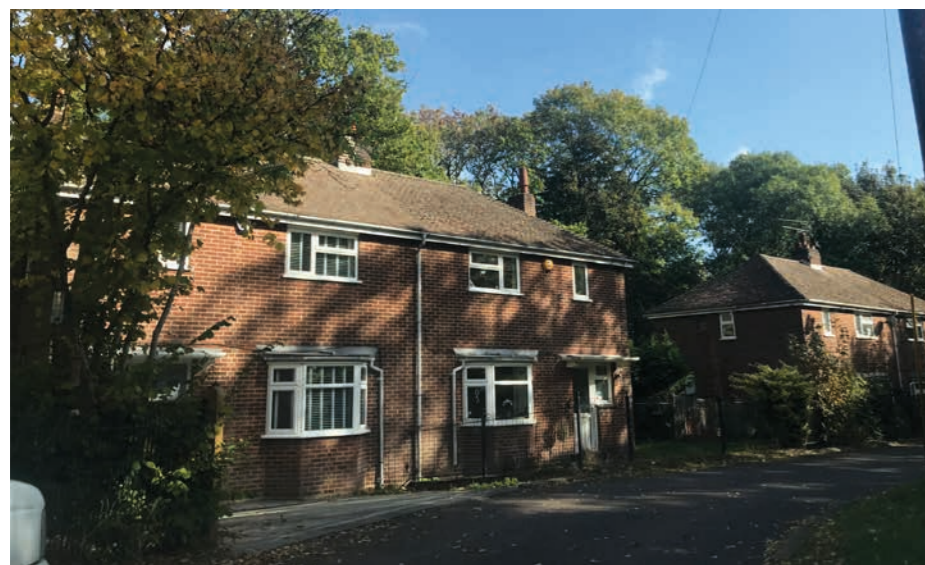
Existing housing along Crow Drive
