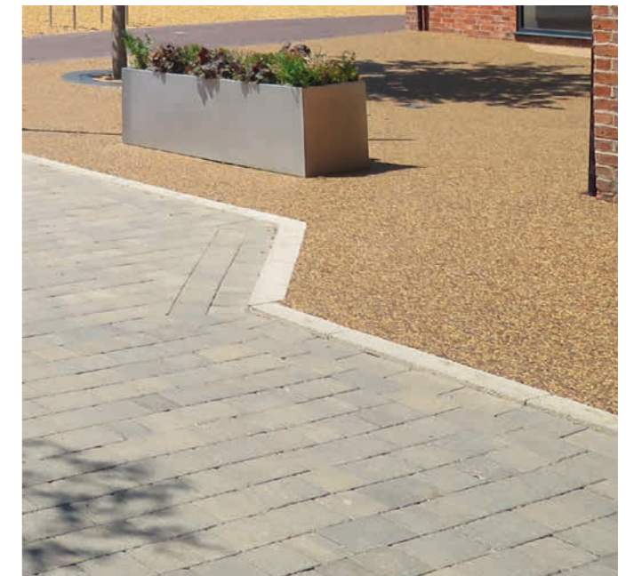
An example of carriageway/shared surface in resin bound gravel and block paving
