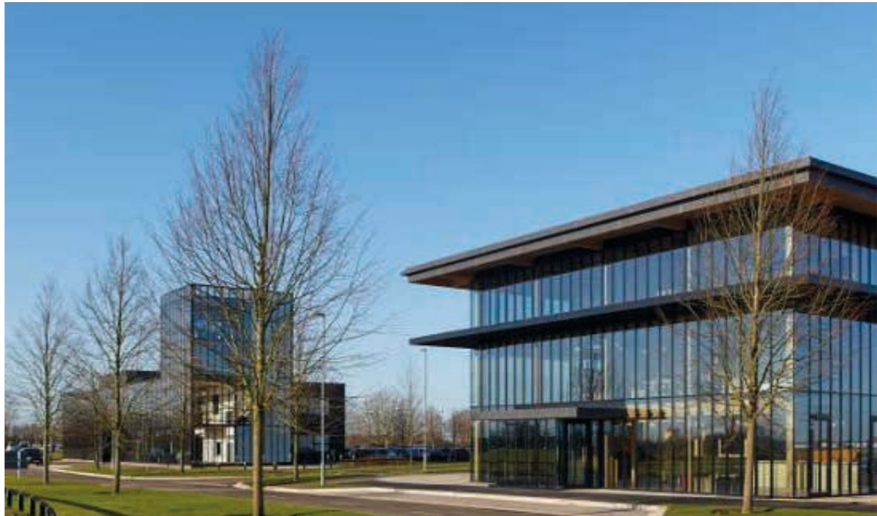
Office/R&D buildings at Alconbury Weald, Huntingdon
