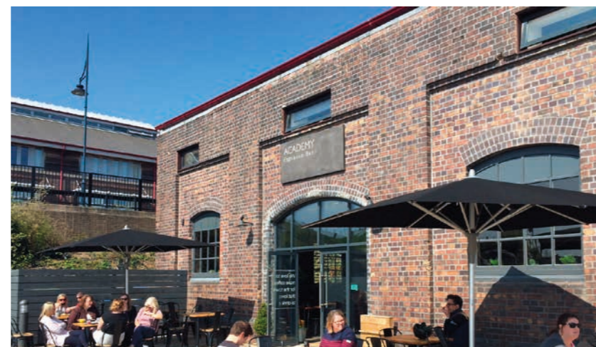
Precedent image of refurbished listed building (Barry, Wales)
