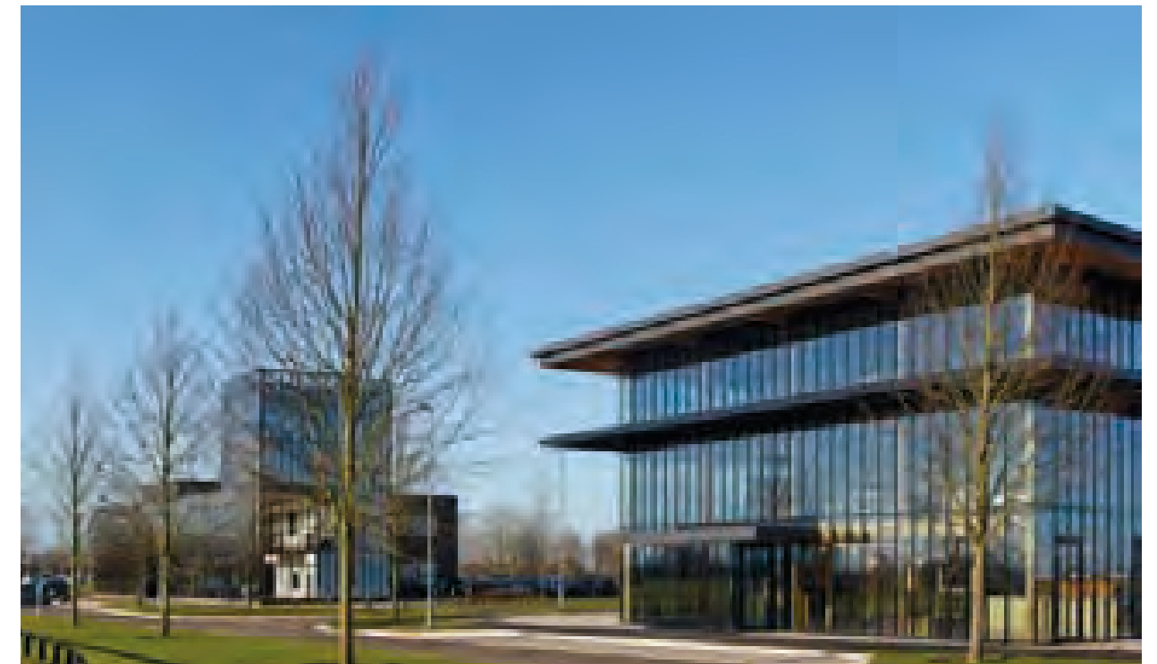
Office/R&D buildings at Alconbury Weald, Huntingdon
