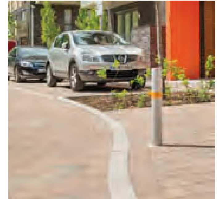
An example of defined parking areas with concrete kerbs and block paving
