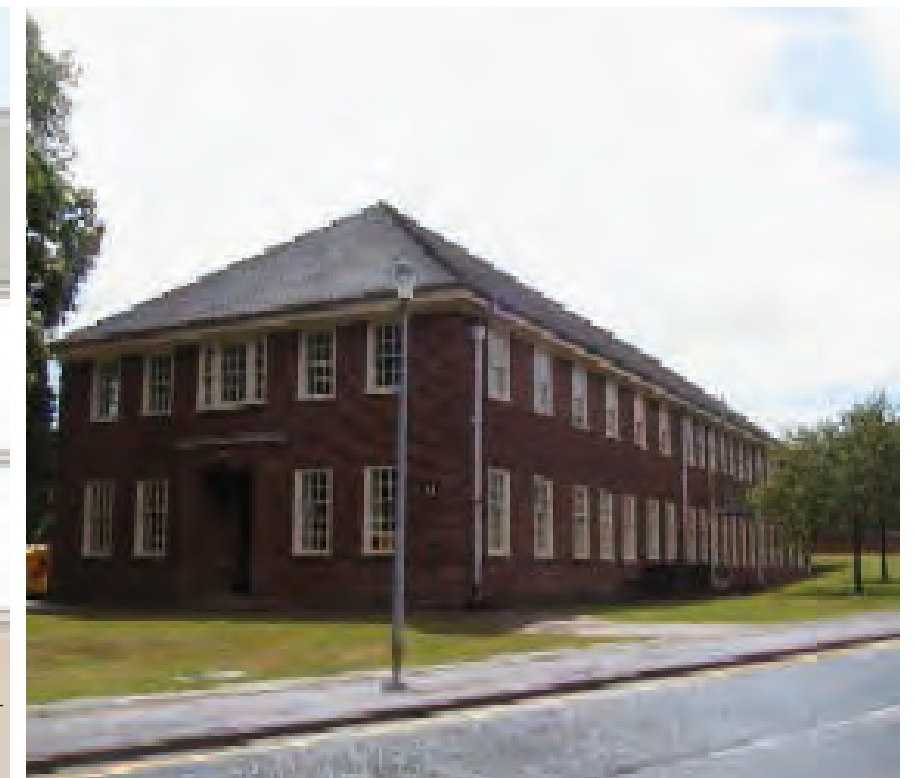
A1 building to be retained
