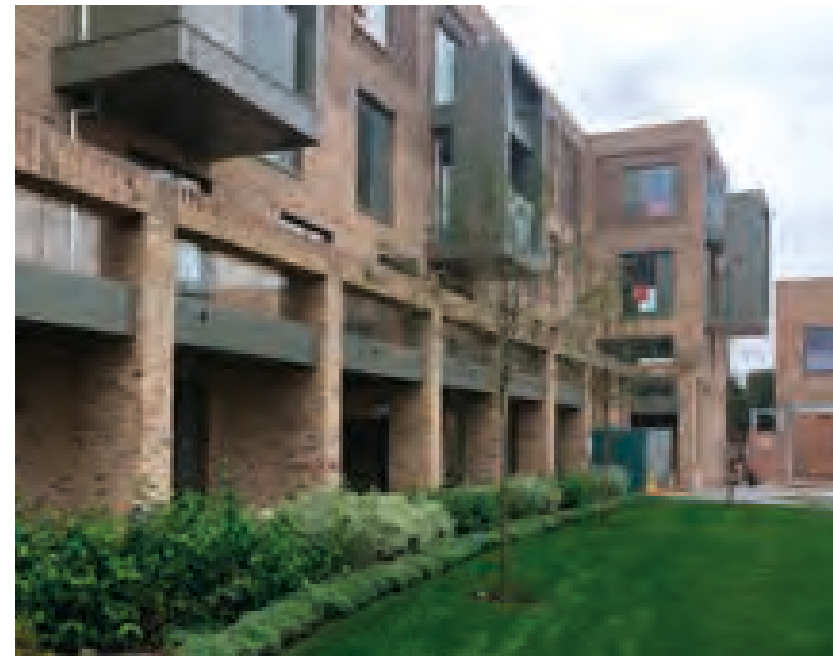
Apartments with ground floor mixed-use (Great Kneighton, Cambridge)
