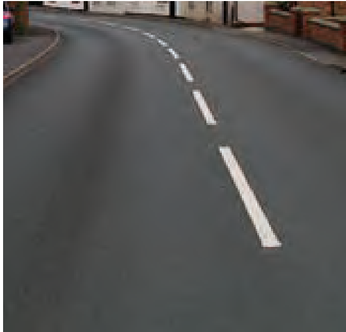
An example of primary roads in asphalt surface
