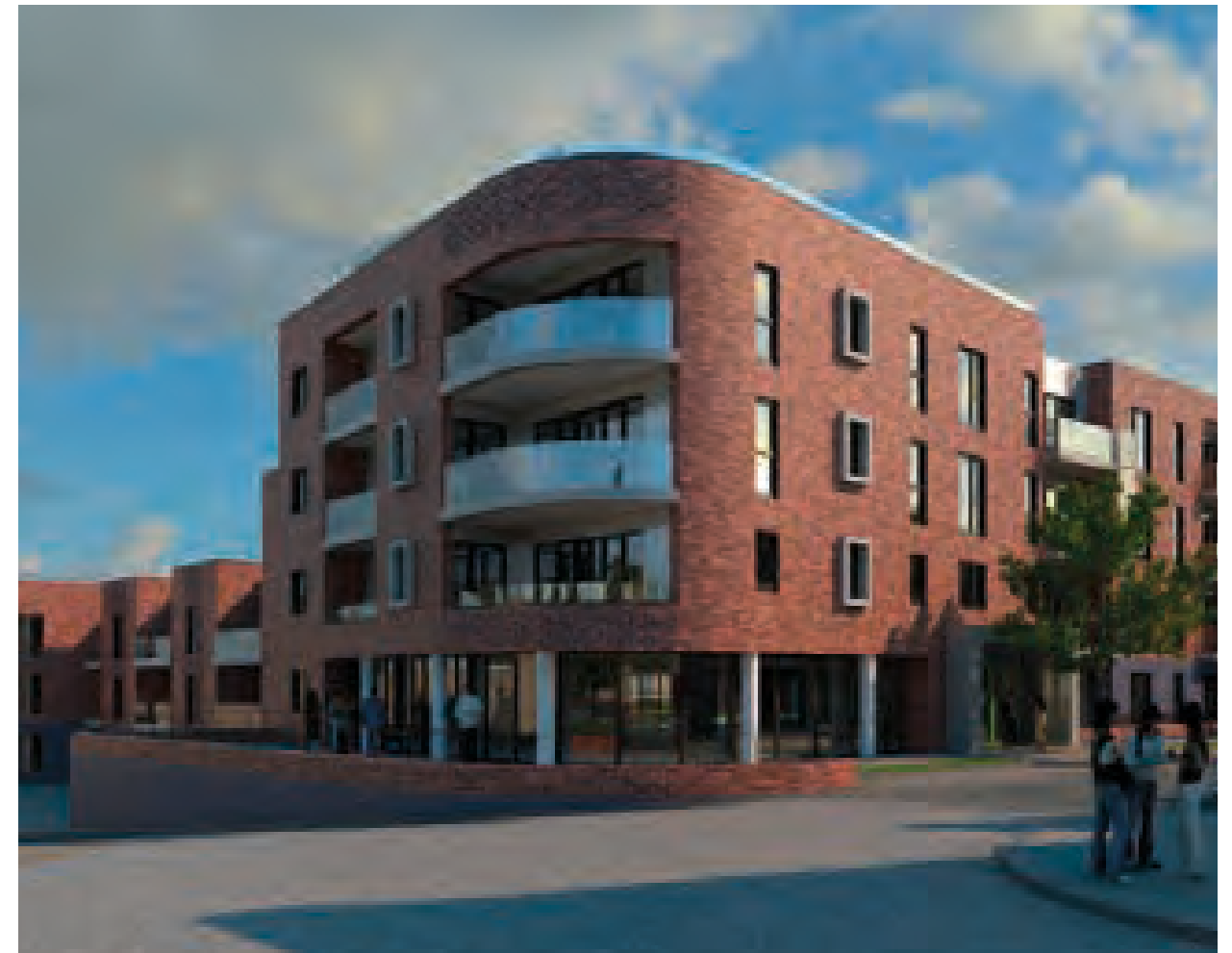
Older people's living accommodation (Lenton Flats, Nottingham)
