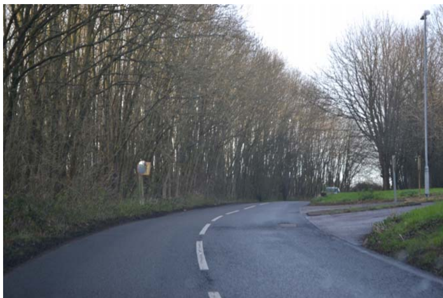
Photo 3: Existing Site Access Junction
