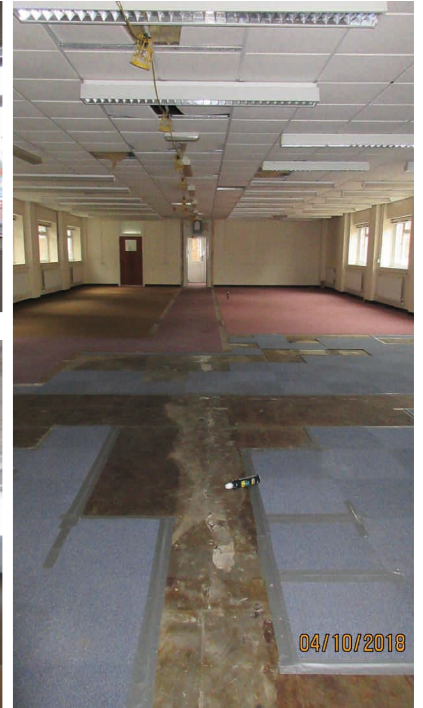
Ground floor / suspended ceiling / blocked window openings on west elevation
