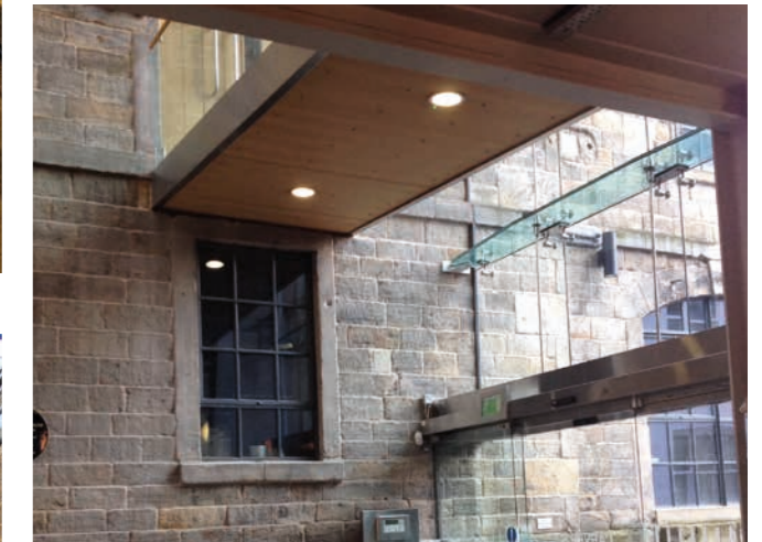
Minimal fixings to existing buildings
