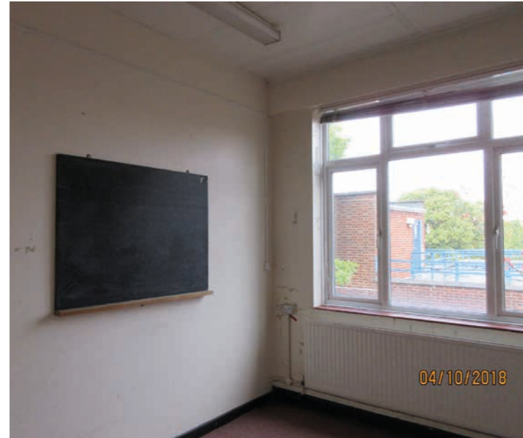
First floor room overlooking Q13
