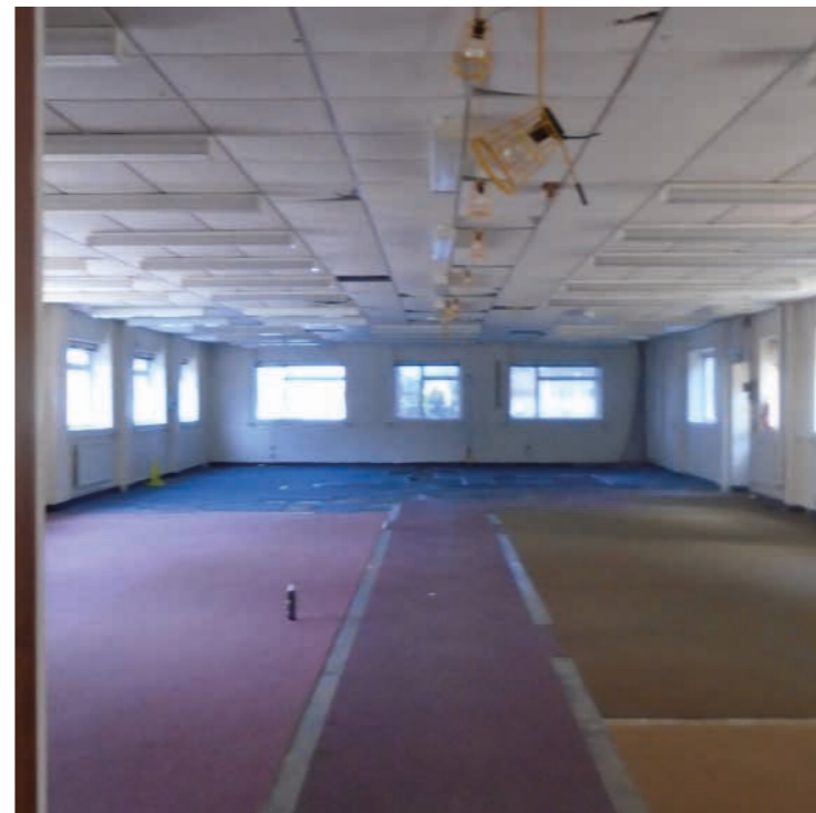
Ground floor / suspended ceiling / blocked window openings
