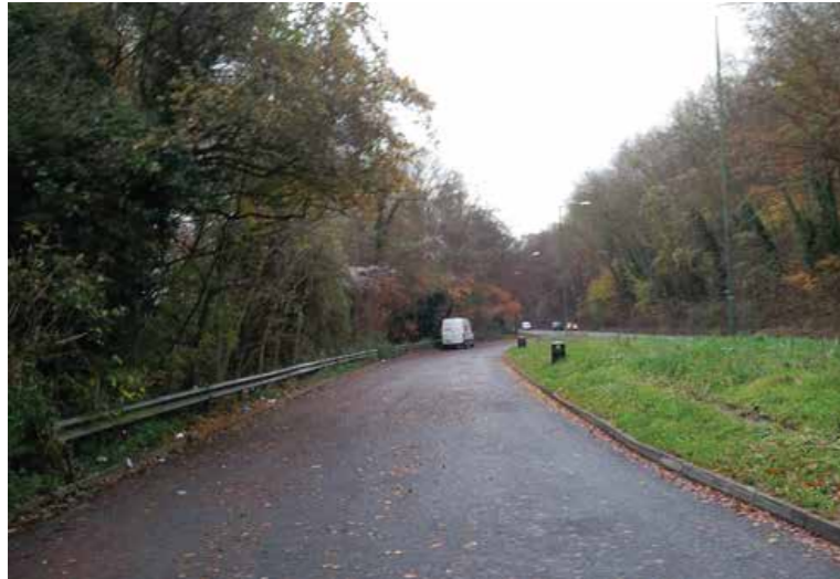
Plate 19d – Slope cutting along A224 to the east of the site (looking southwest).
