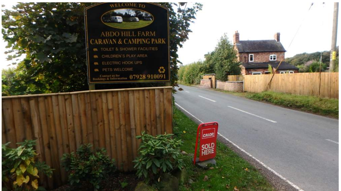
PHOTOGRAPH 2 Visibility splay @ 2.4m to the left (south)
