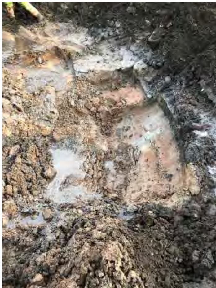
Photo 2: Natural Soils Below Former Underground Tanks
