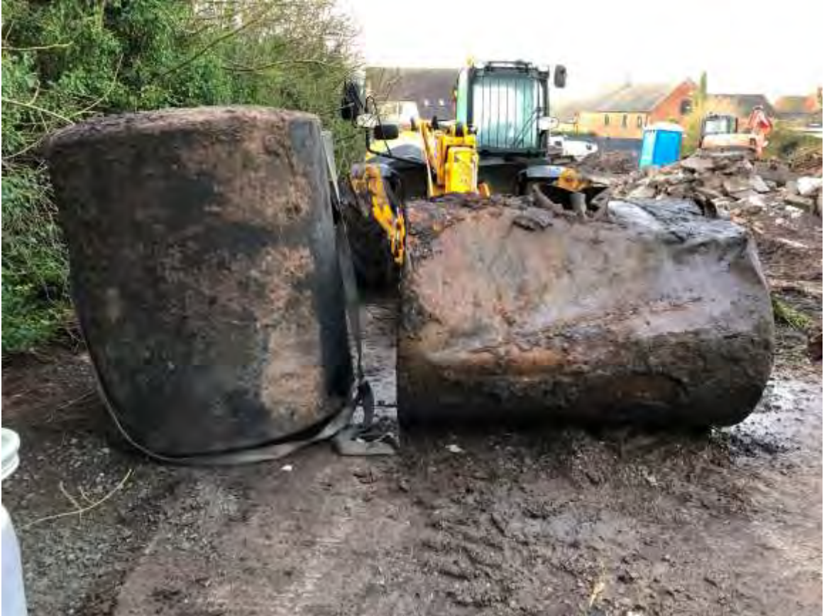
Photo 1: Excavated Underground Tanks Awaiting Off-Site Disposal
