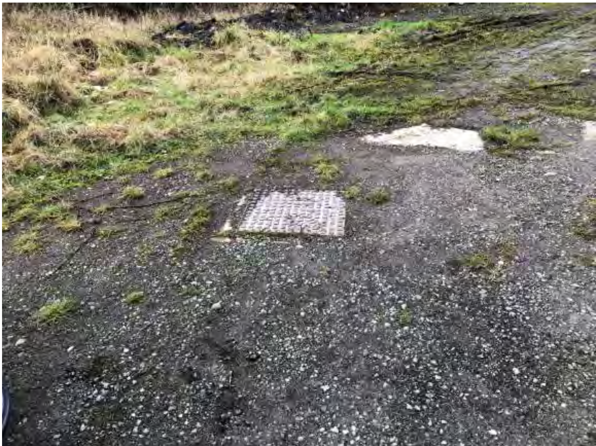
Photo 6: Existing Manhole Cover
