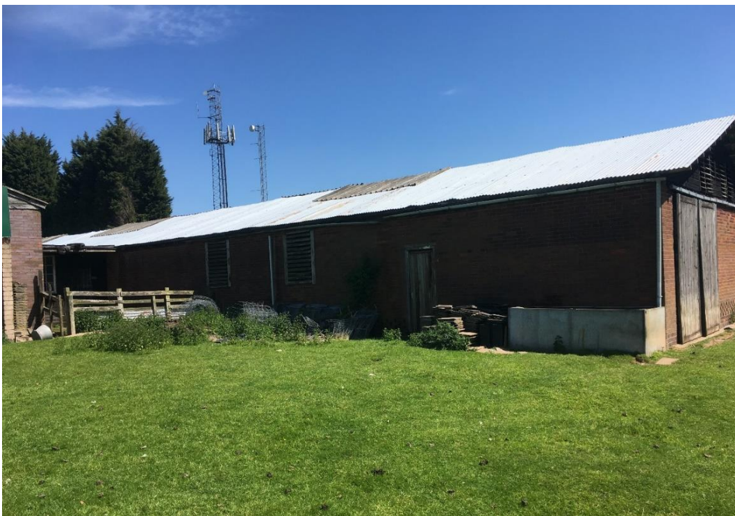
Photo 3.2: The agricultural building for conversion (west elevation)
