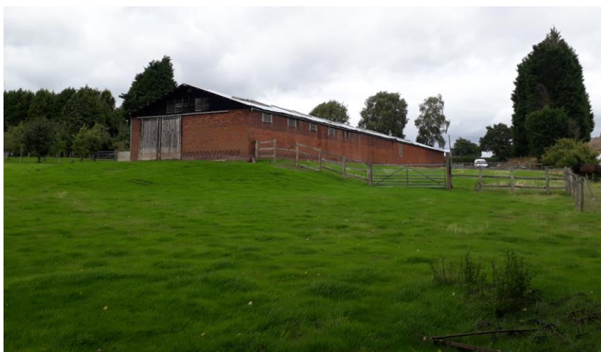
Figure 6 Brick built agricultural building proposed for residential conversion.
