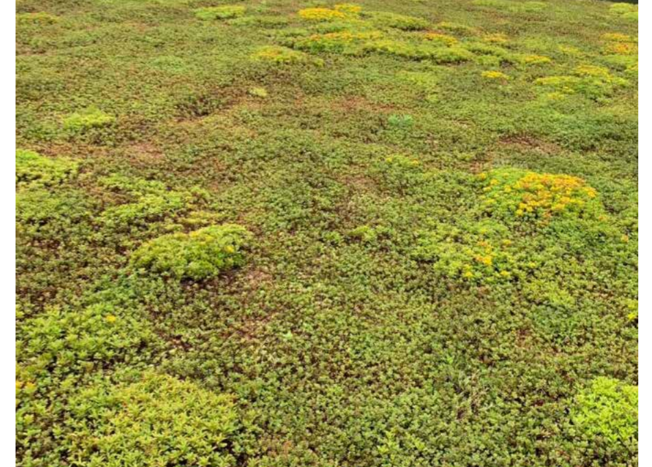
Planted Green Roofing
