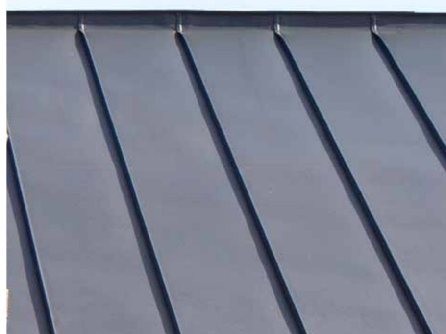
Metal Standing Seam Roofing
