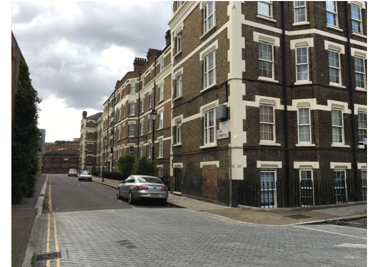
Figure 3.11: View due west along Cons Street from Greet Street, with the Ipsden flats in the foreground.
