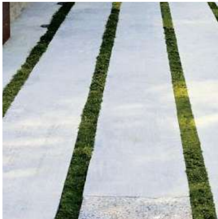
Concrete plank paving to footpath
