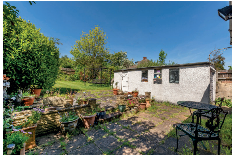
Fig.5 View of the existing garage/workshop
