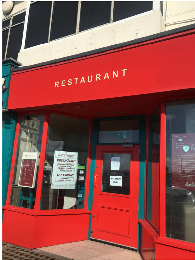
Ph02 Existing restaurant entrance on Marine Parade
