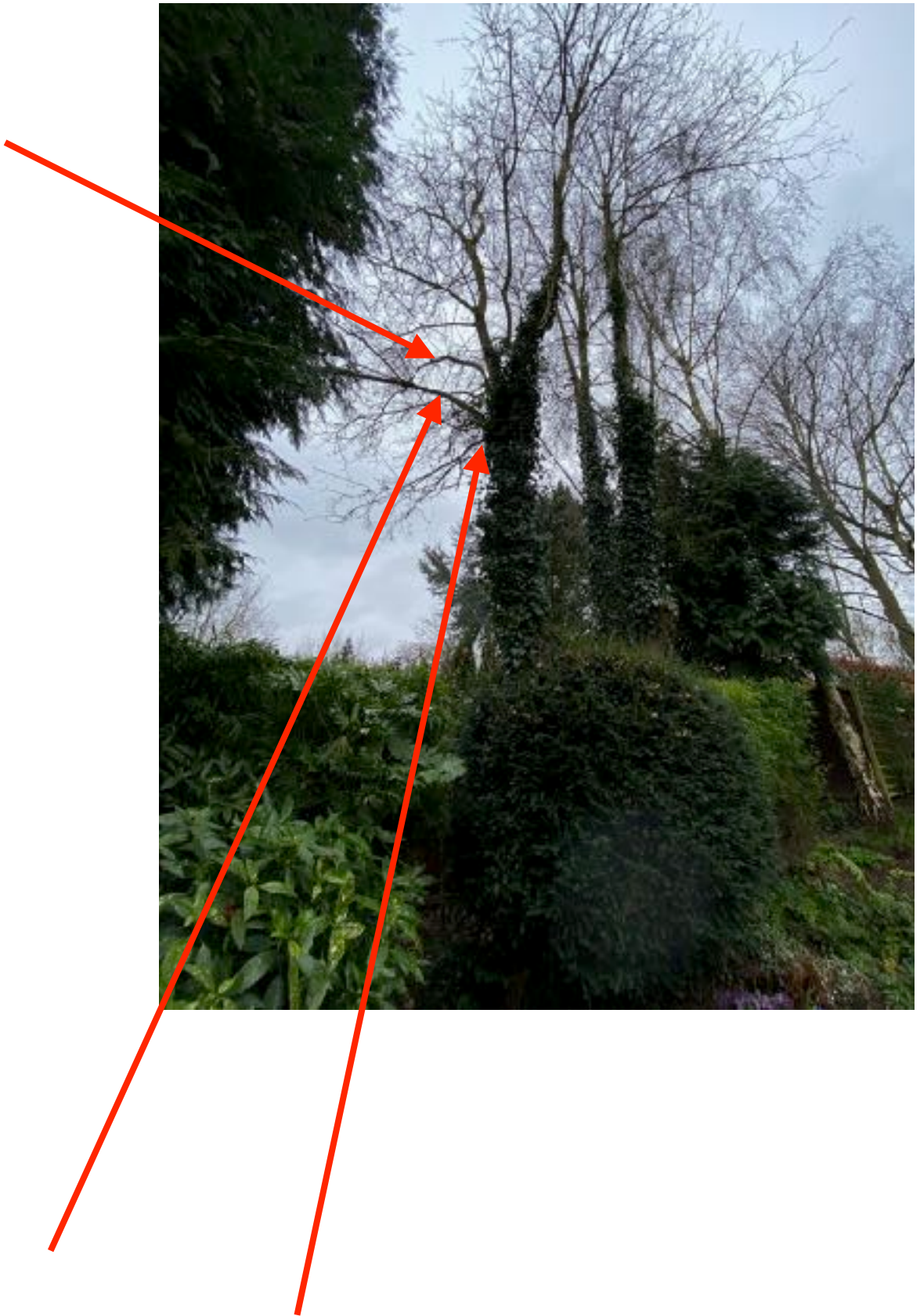
T1 - Red arrows show the 3 branches that over extend into the neighbouring property. Approximate length of branches is 4m.
