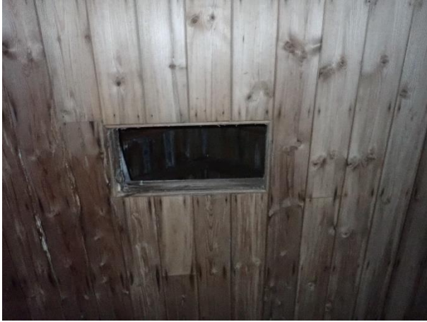
Well spaced wood sarking present
