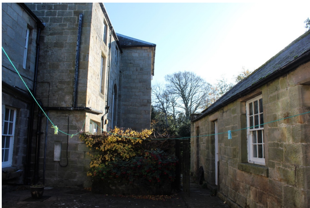
The outbuildings and north elevation
