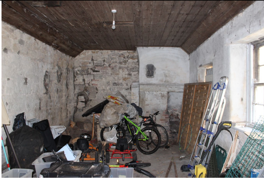
North wall, proposed studio with blocked fireplace and concrete floor.
