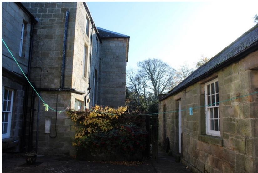
The east elevation of the outbuildings looking south
