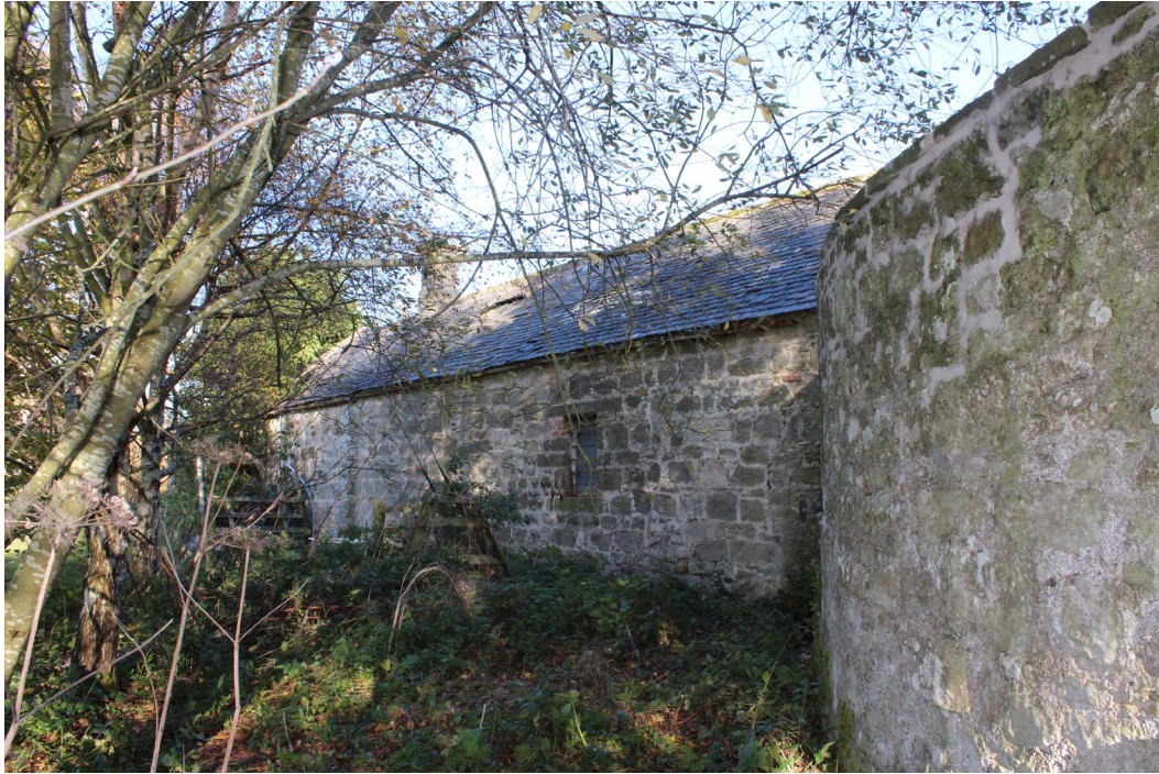
The outbuilding west elevation
