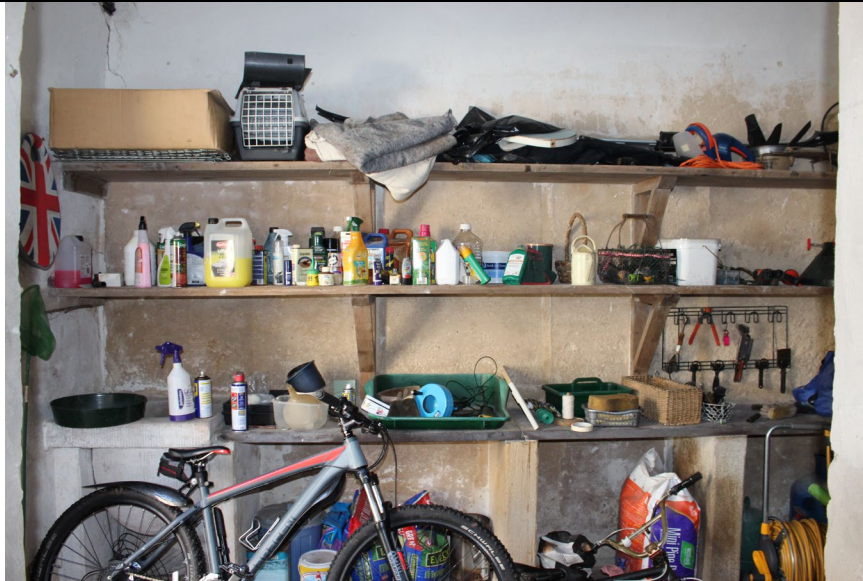
Existing store room with stone shelving which will have a section removed to form an opening for access, but the remainder of the shelving and stone bowl retained.
