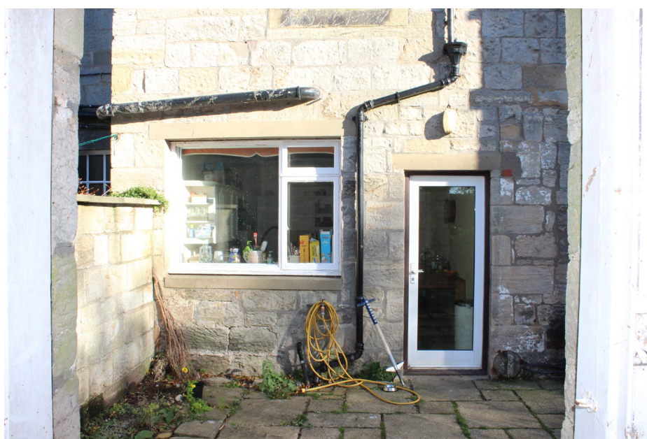
Existing west elevation modern openings
