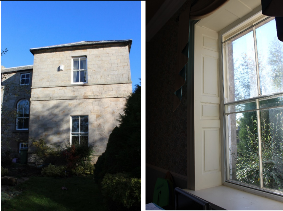
West elevation with window to be removed and opening altered to form opening to the garden room.
