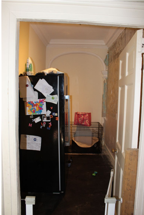
Existing hallway/ proposed location of new wc.
