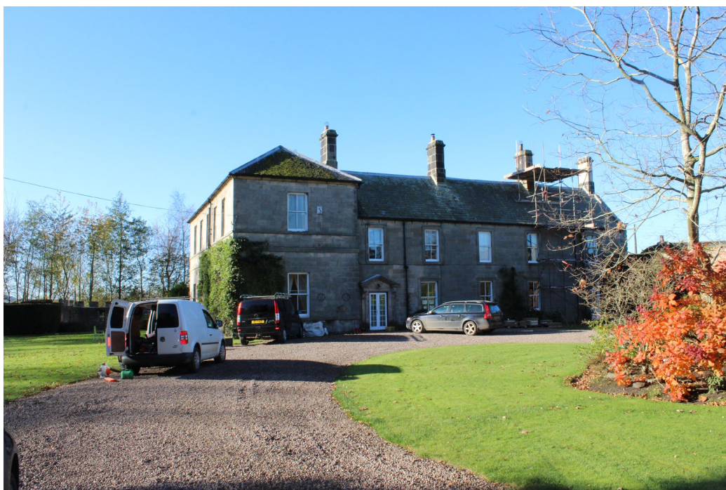
The main approach to Bolton Hall from the east, note the north hall adjoining to the right
