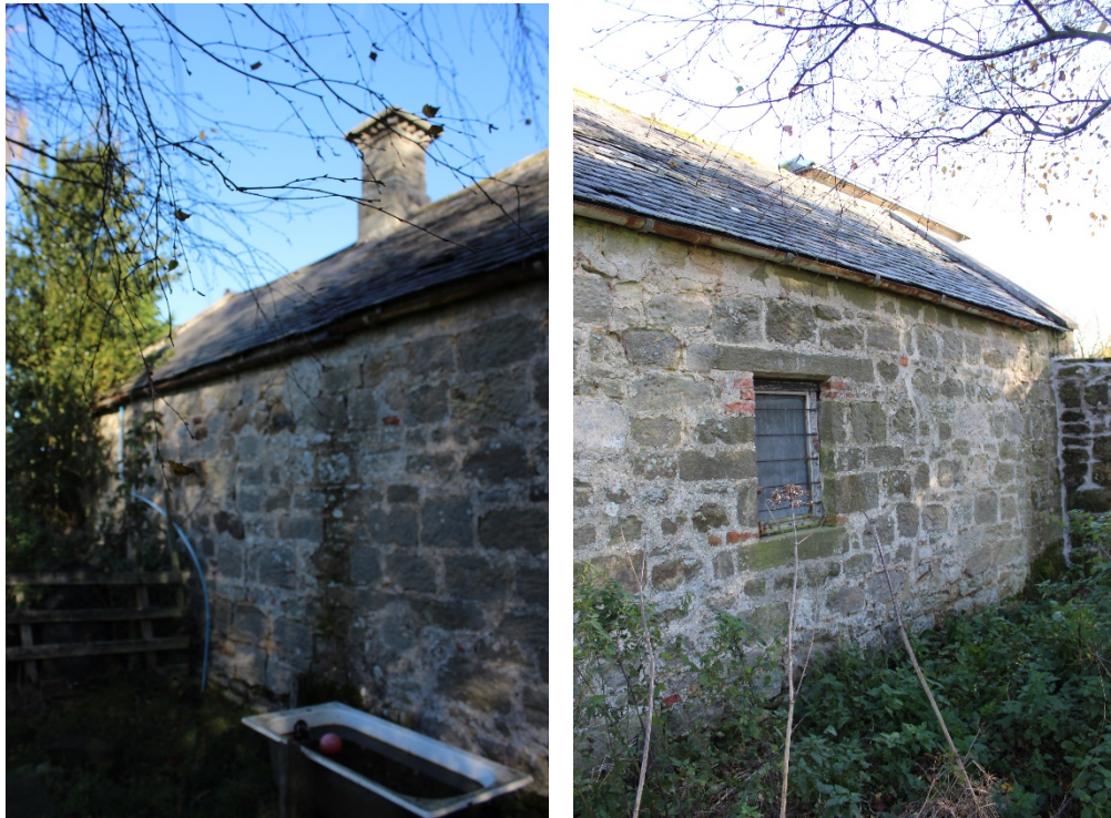
The outbuilding west elevation
