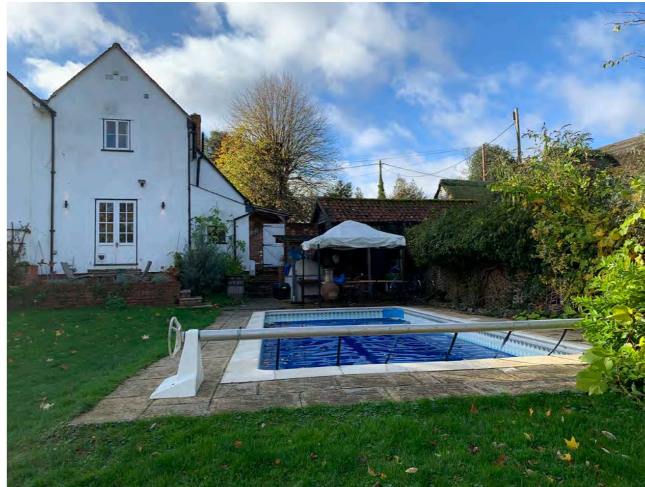
Existing view of the Swimming Pool
