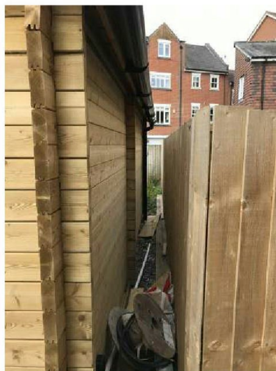
rear of outbuilding 2
