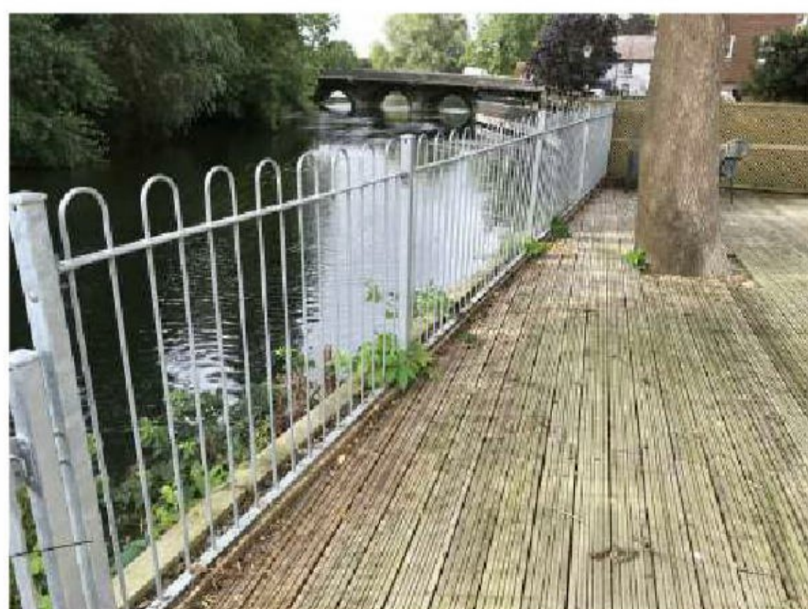
view from decking looking south towards bridge
