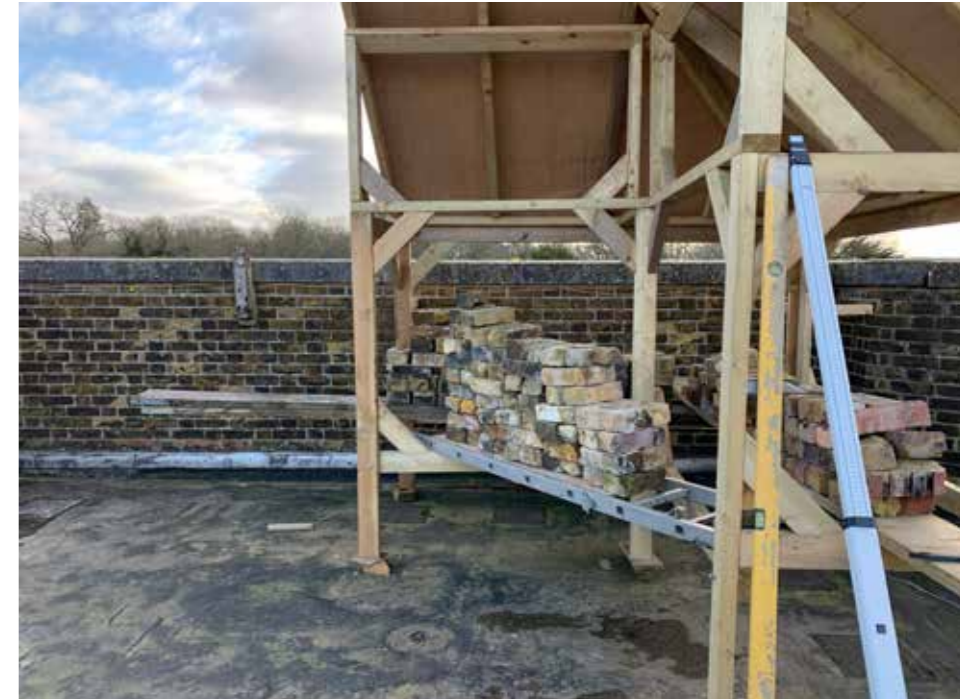
Plate : 34 Parapet and temporary roof mock up.
