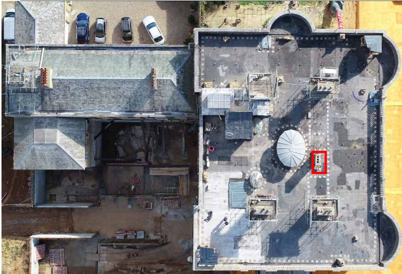
Plate 2: Above: Aerial view taken in October 2018 The non-original chimney highlighted in red is to be relocated centrally.
