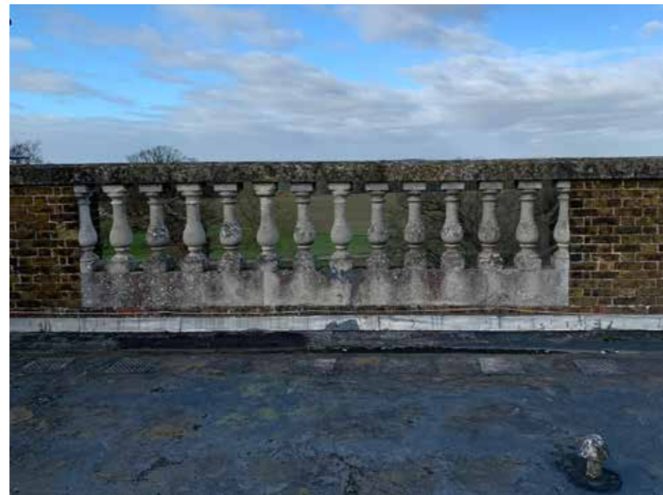
Plate : 21 Parapet and Bottle balusters
