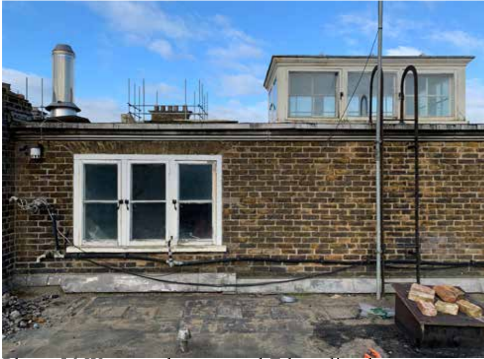
Plate :56 Water tank room and Edwardian lantern (from East)
