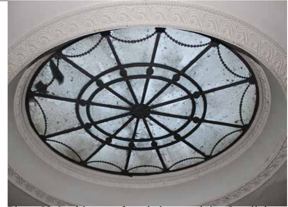
Plate :58 Oval lantern from below retaining Lay light and cornice detail.
