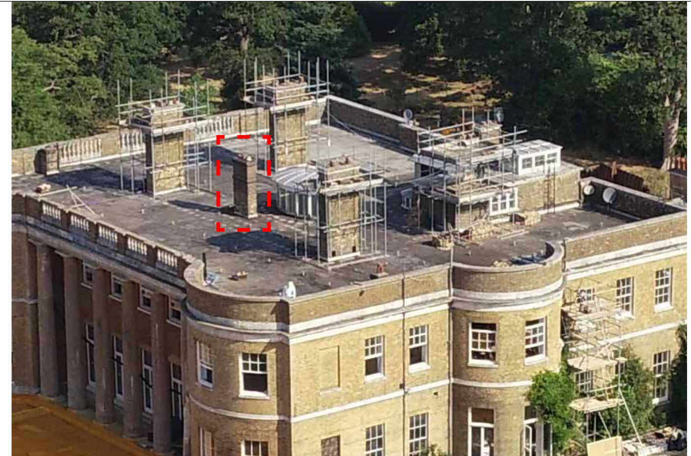
Plate 3: Above: Photo of Sacombe House roof taken in 2017 the chimney which is to be relocated is highlighted in red.
