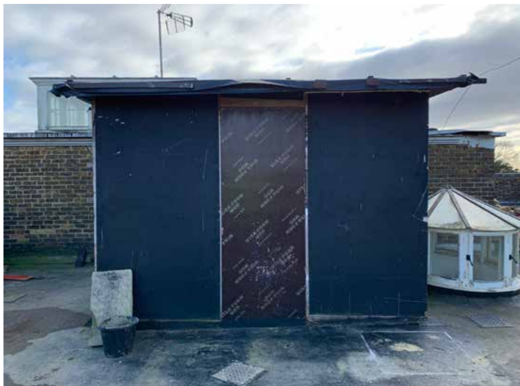
Plate : 49 Top of Service lift shaft
