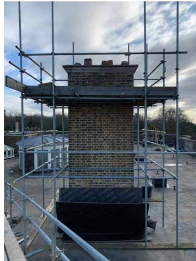
Plate :54 South-west Chimney stack to be raised above new consented roof and new Georgian pots to be added
