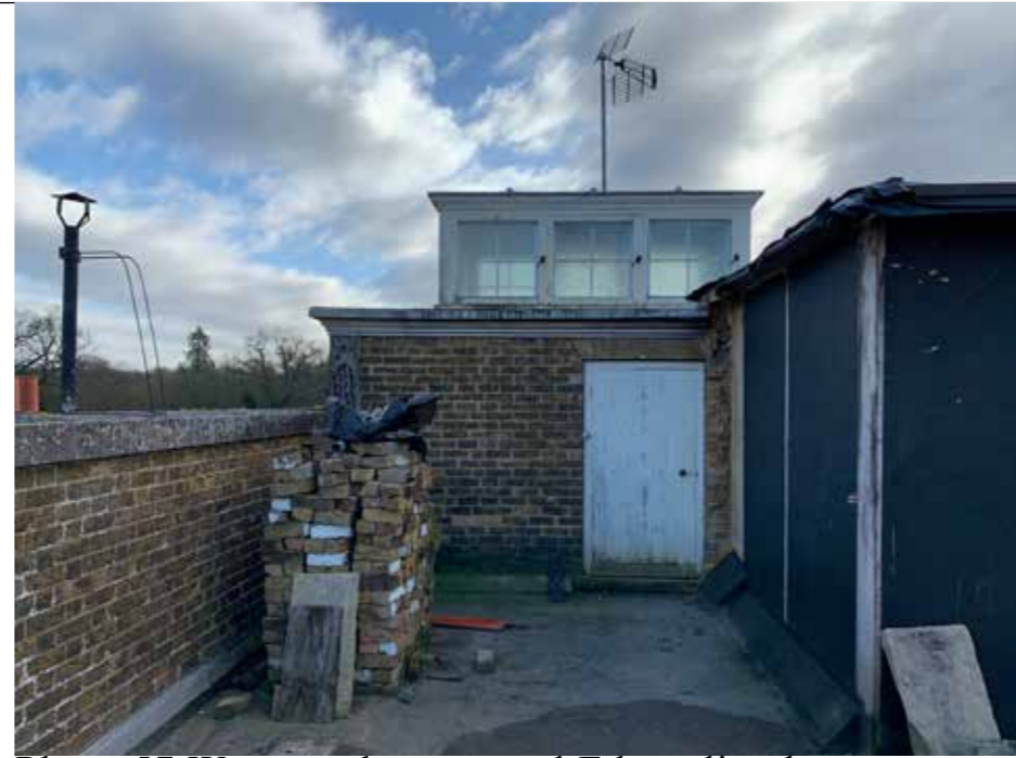
Plate :57 Water tank room and Edwardian lantern (from West)
