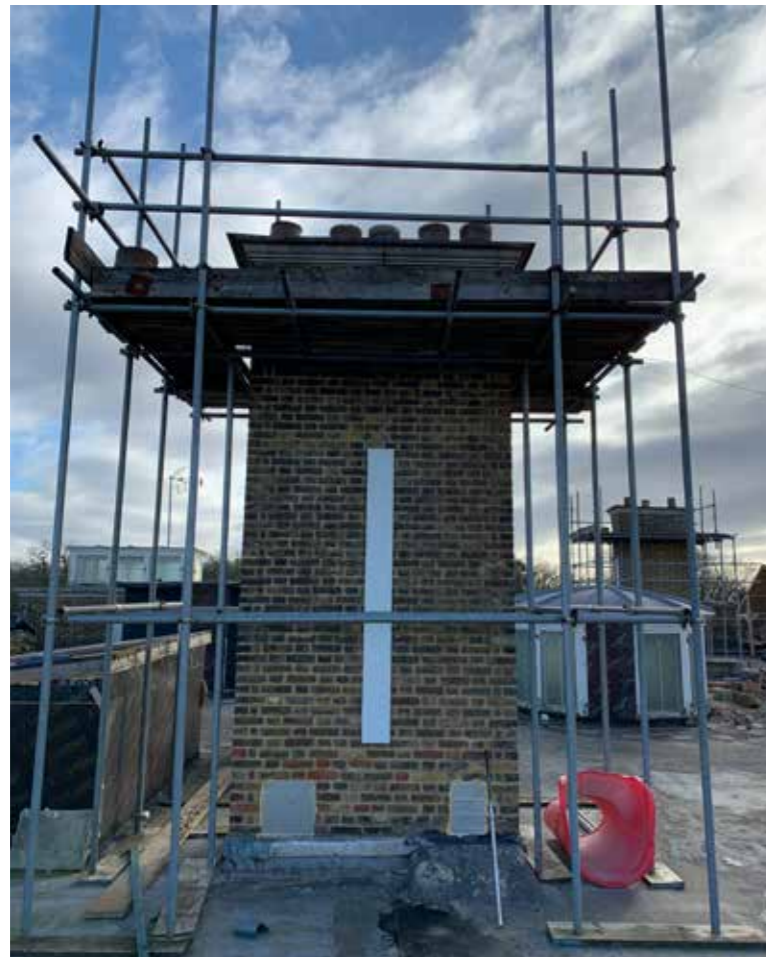
Plate :53 North west Chimney stack to be raised above new consented roof and new Georgian pots to be added
