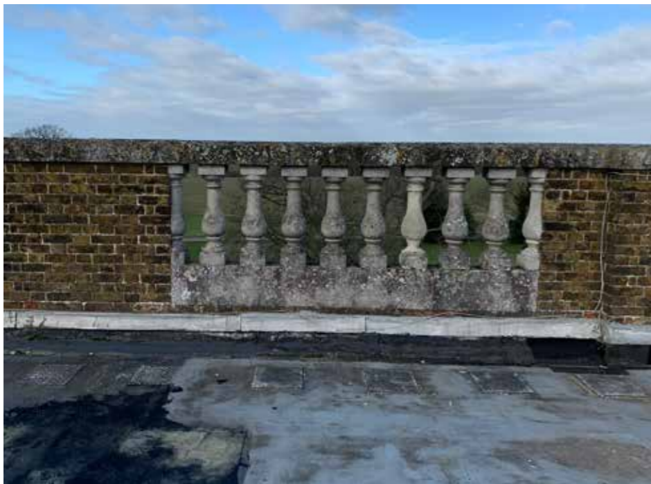
Plate : 20 Parapet and Bottle balusters
