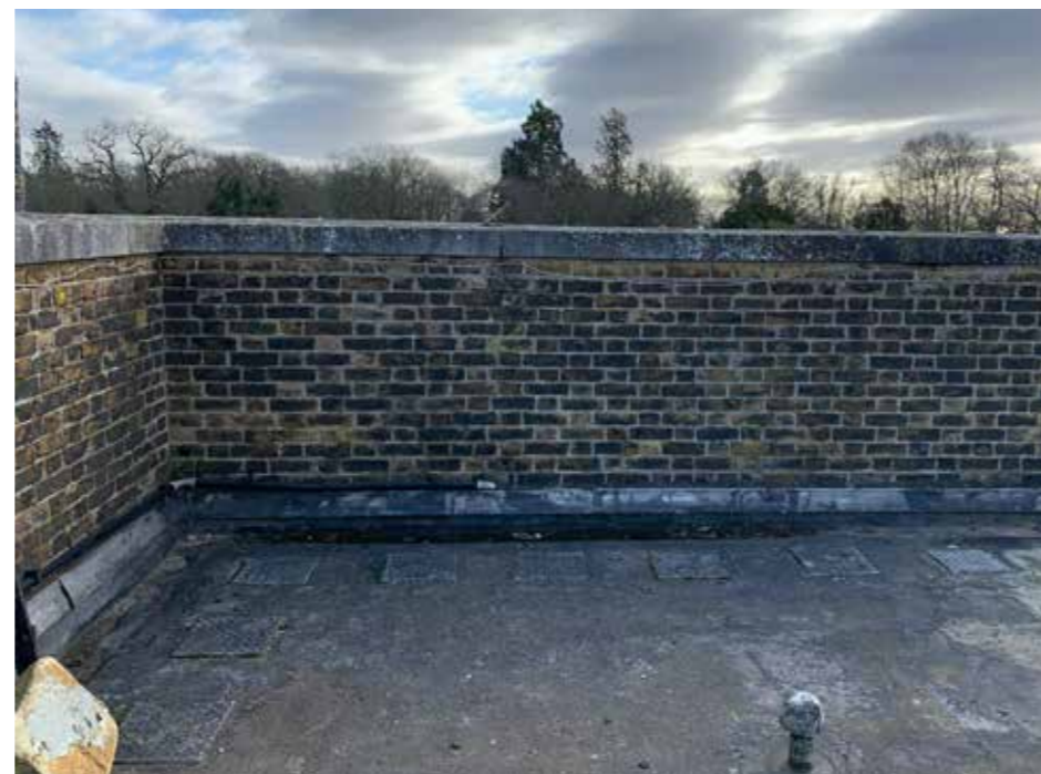
Plate : 39 North east corner of the parapet.
