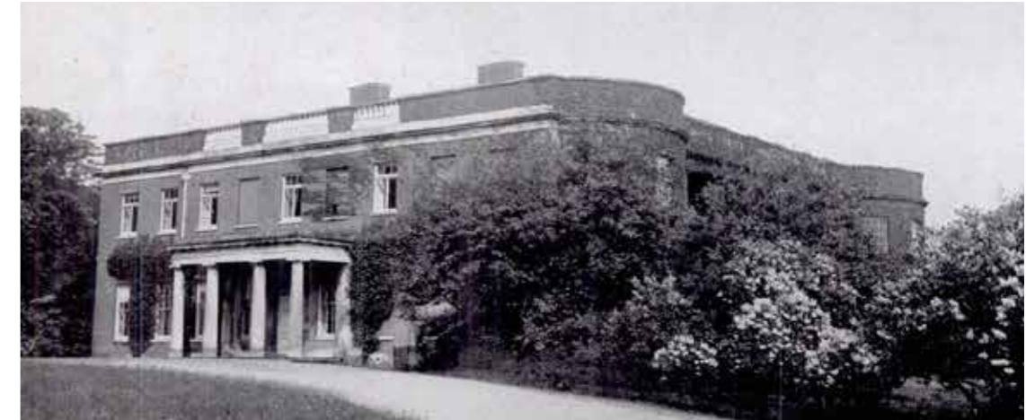
This photograph, found in Country Life Magazine issue 09 and taken in 1936, shows the chimney stacks having been rebuilt to a lower height with no pots.
