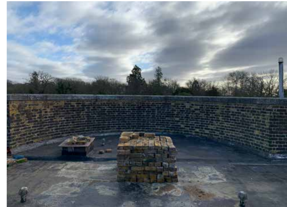
Plate : 37 Curved Parapet over eastern bay.
