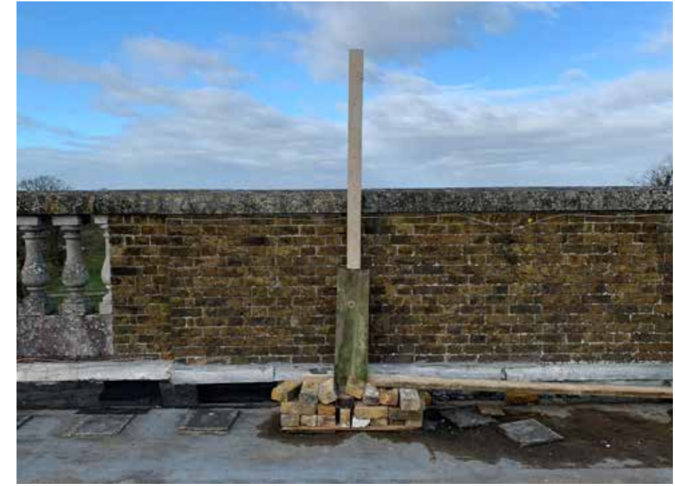
Plate : 19 Western parapet and existing Bottle balusters
