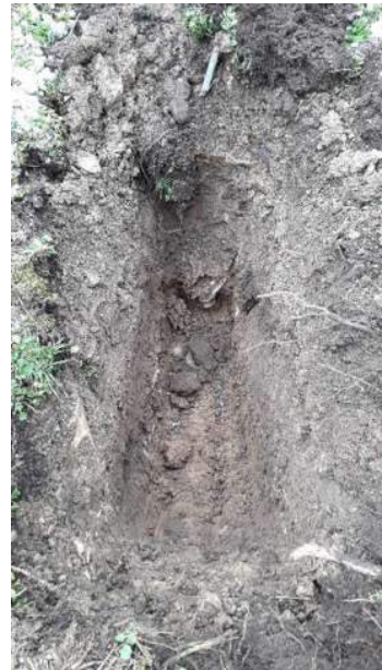
TP05: with groundwater beginning to seep in at the base
