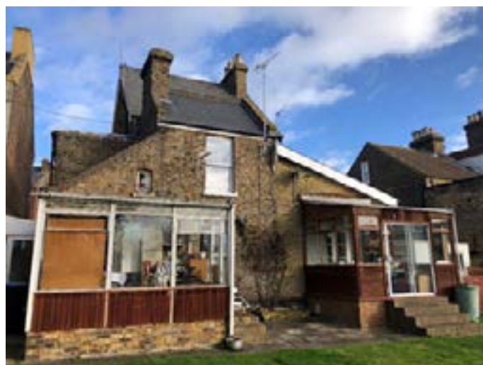
Figure 3: Photograph of rear elevation of No. 11 Ellington Road
