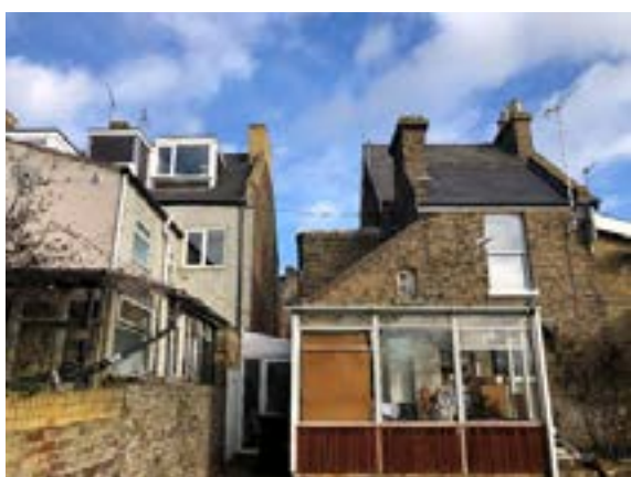
Figure 9: Photograph of rear elevation of No.11 & No.13 Ellington Road
