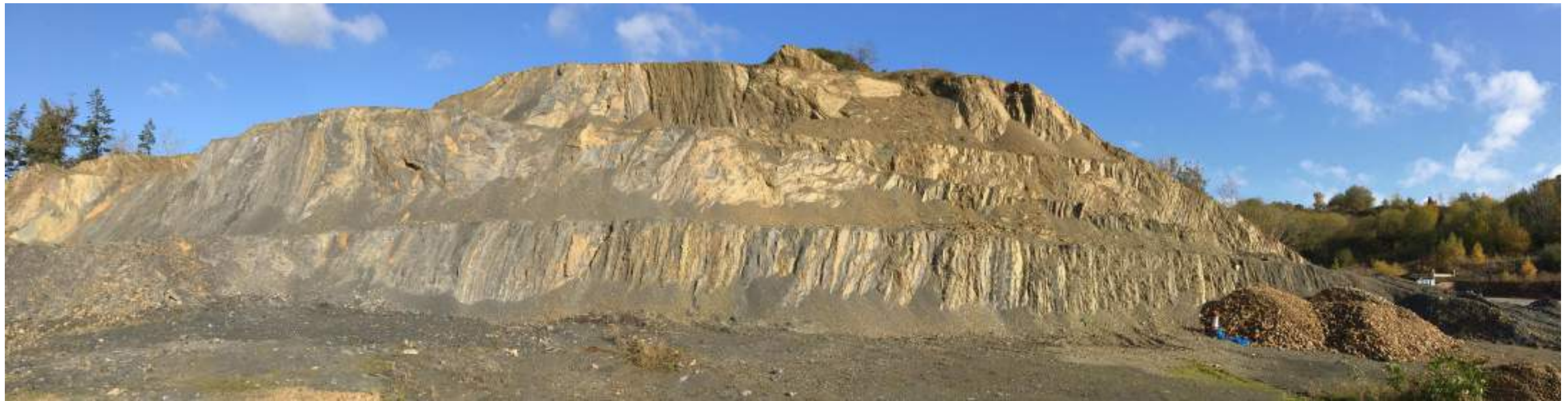
Photograph 1: Panoramic view looking northeast of existing excavation southwest facing benches located approximately 90m north of weighbridge office. Generally sub-vertically bedded interbedded shales and sandstones of the Cefn Formation. Note faulting in the upper slope which has resulted in planar surface dipping out of the slope at approximately 45°. Note presence of spalled material at base of each face which is fine grained; silt to coarse sand sized matrix with some gravel. Overall face is dry with no indications of groundwater seepage.
