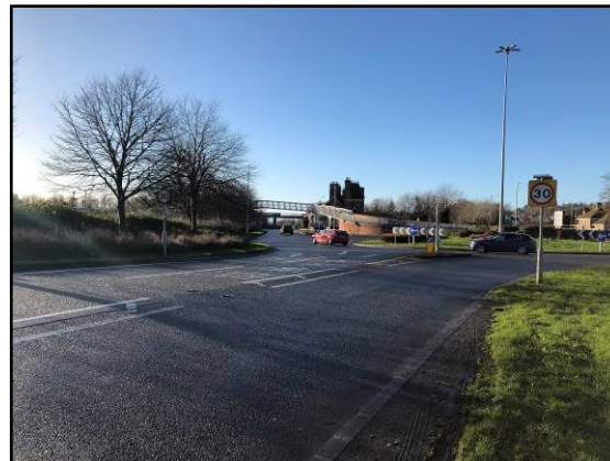
Plate 4: A view of the A483 / B4381 / Smithfield Road Roundabout
