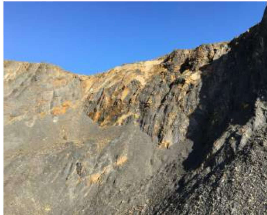
Photograph 3: Possible fault zone present in lower face or northern excavation.
