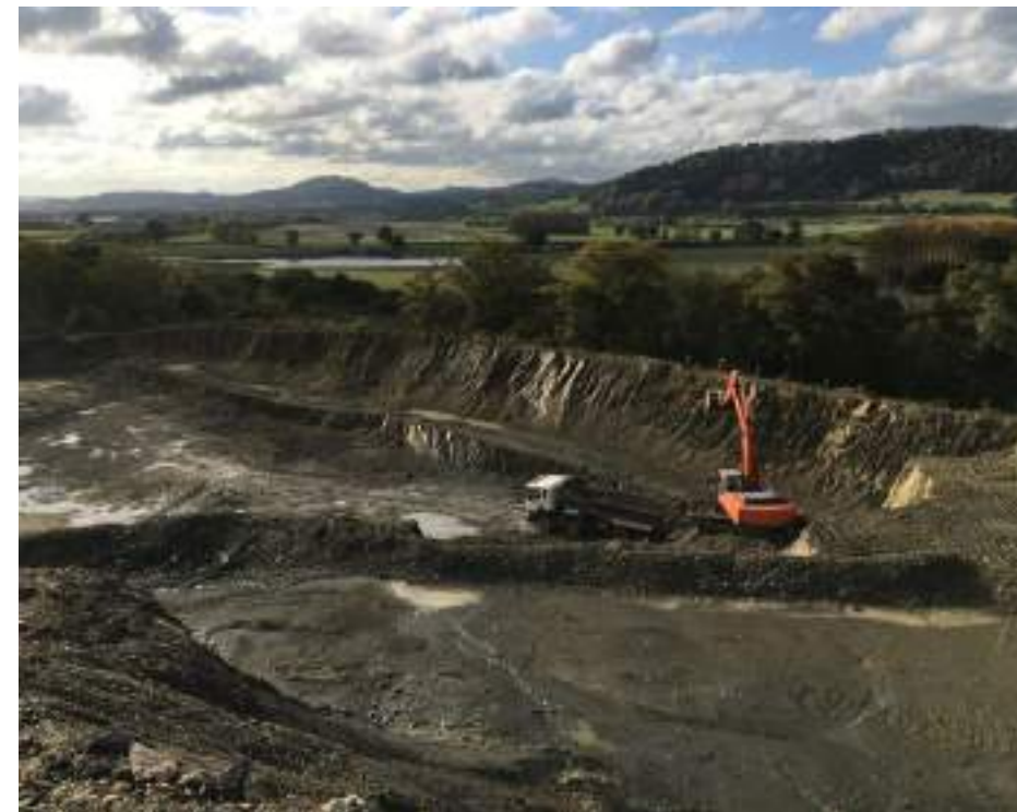
Photograph 13: View looking southwest showing overview of western excavation face.
