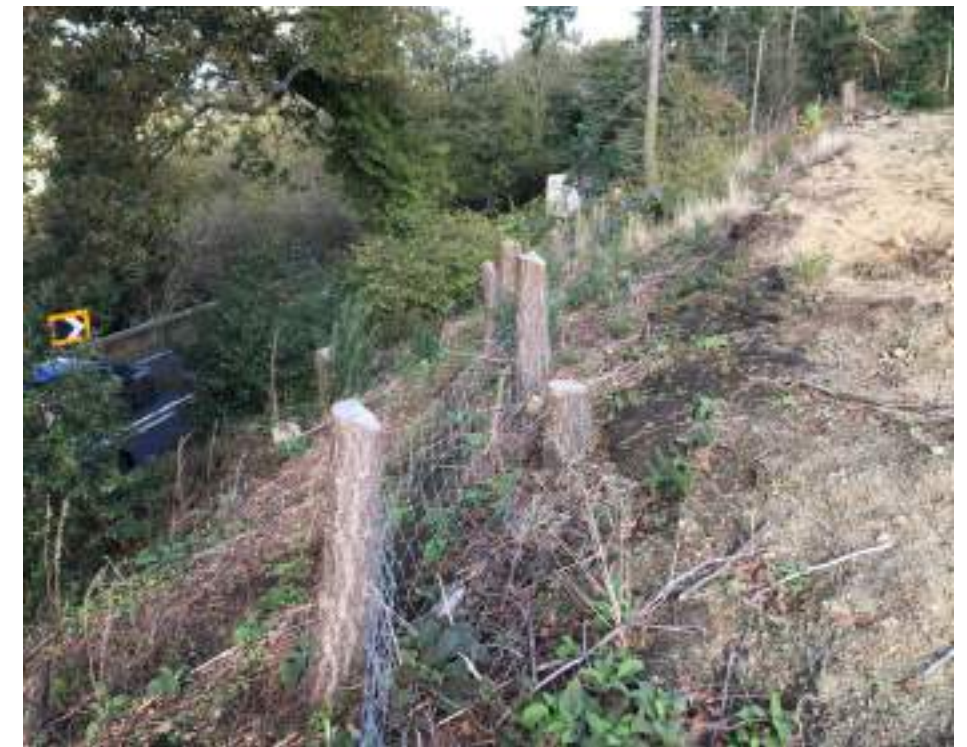
Photograph 11: View looking northwest of slope leading down to A458 showing steep slopes partially cleared of trees.
