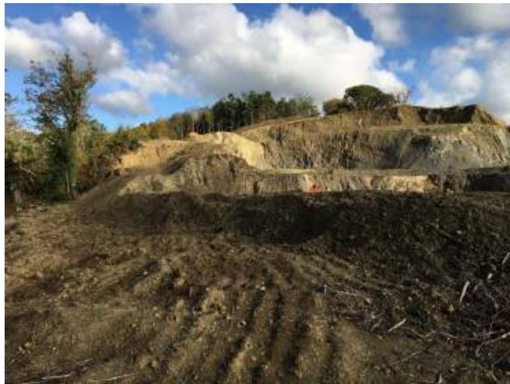
Photograph 9: View looking northeast of upper excavation faces.
