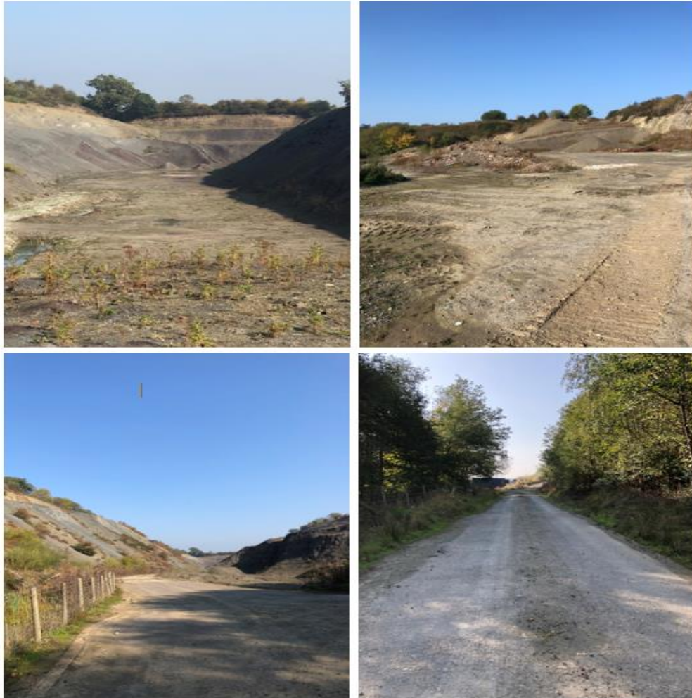
Figure 5-1: Development Site Character
