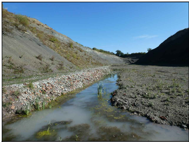
1. Pounded water in quarry floor drains to South-West
