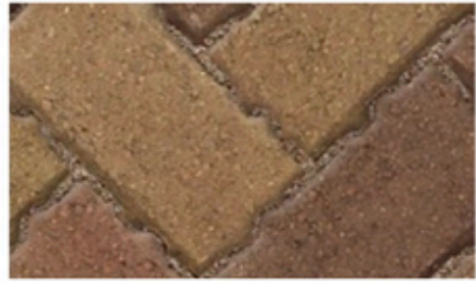
Brick pavers for shared surfaces
