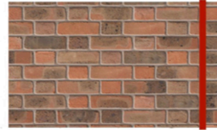
Flemish bond brick wall at entrance
