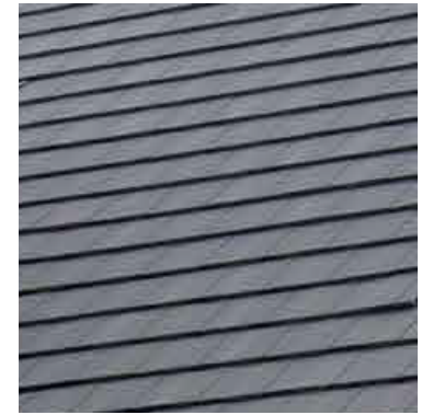
Roof: Redland Landmark 10 Slate in Brecon Grey
