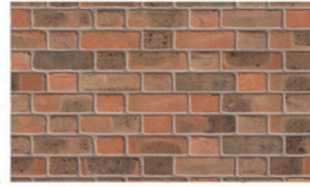
Flemish bond brick wall at entrance
