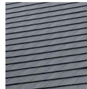
Roof: Redland Landmark 10 Slate in Brecon Grey
