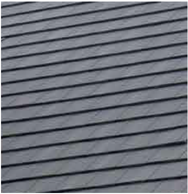
Roof: Redland Landmark 10 Slate in Brecon Grey
