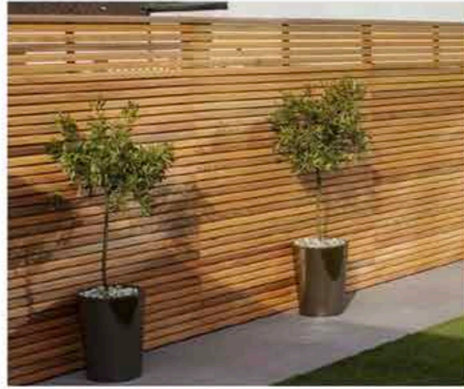
Horizontal fencing between house plots
