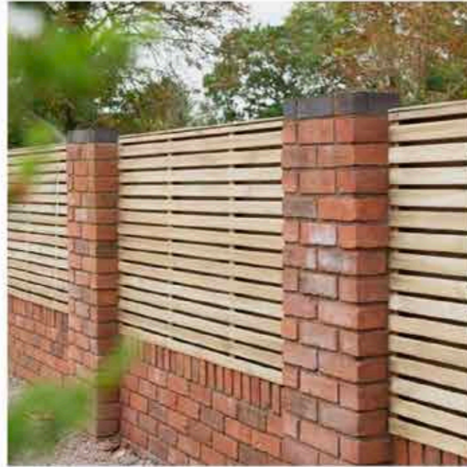
Brick base and pillar with horizontal fencing
