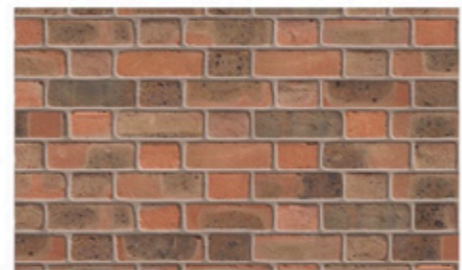
Flemish bond brick wall at entrance
