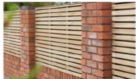
Horizontal fencing with brick piers and base
