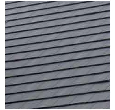
Roof: Redland Landmark 10 Slate in Brecon Grey
