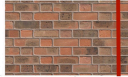
Flemish bond brick wall at entrance
