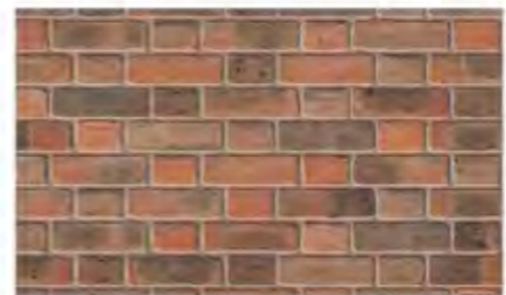
Flemish bond brick wall at entrance
