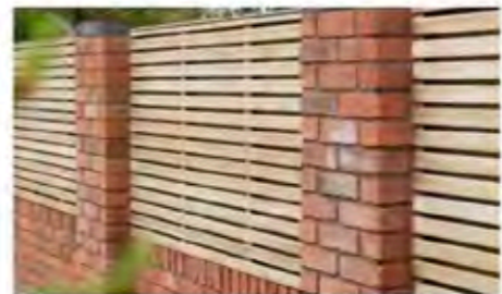
Horizontal fencing with brick piers and base
