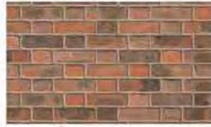
Flemish bond brick wall at entrance
