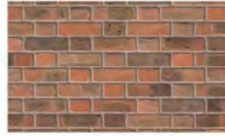
Flemish bond brick wall at entrance
