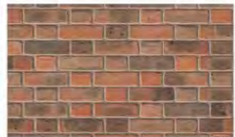
Flemish bond brick wall at entrance
