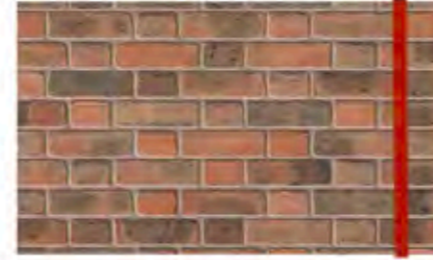
Flemish bond brick wall at entrance
