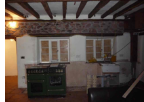
Exposed masonry above north east wall of Kitchen
