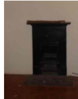
Fireplace in Bathroom 1
