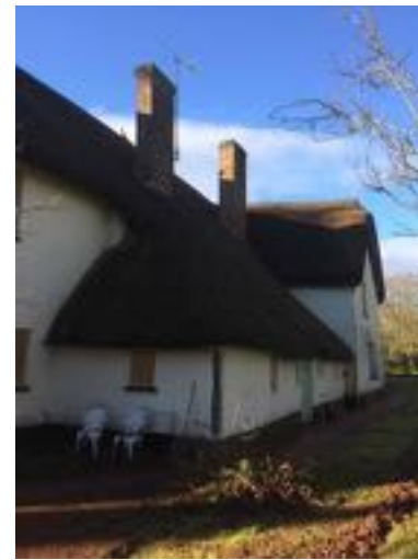
North eastern view of Out Shut to Farmhouse
