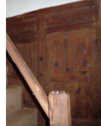
Late 18C panelling used as cupboard doors in Kitchen
