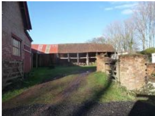
Linhay from the south east
