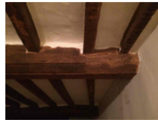
Kitchen ceiling joists socketed into beam.
