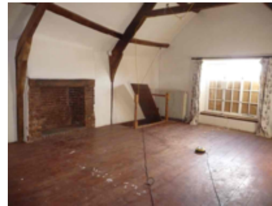
Bedroom1 with exposed trusses
