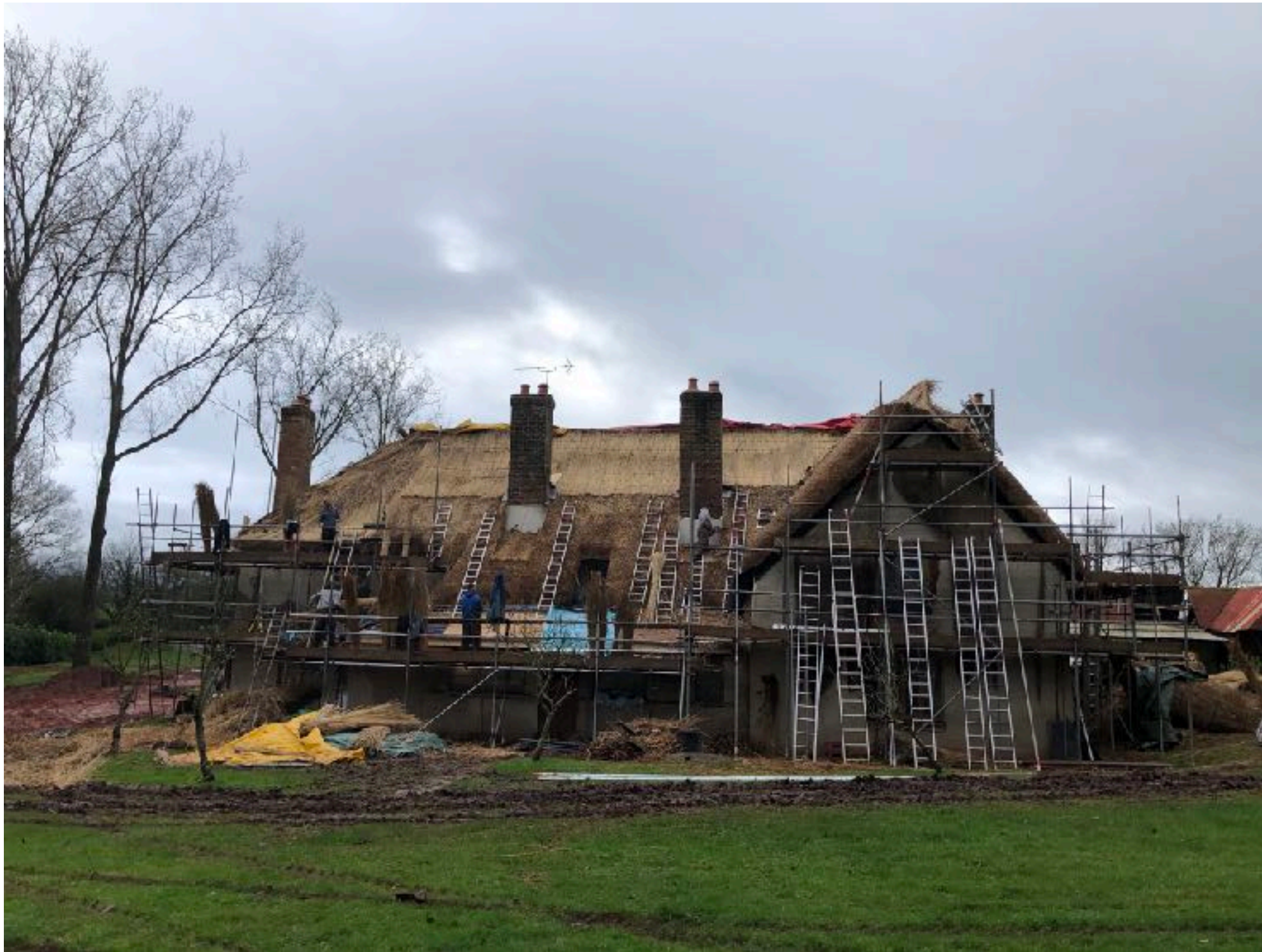
Thatching work in progress December 2020
