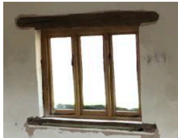
Now: New three light oak framed window and cill installed in place of previous window, leaded casements retained on
