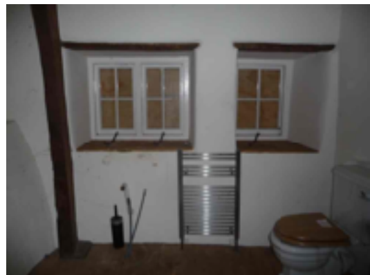
Bathroom 2, north west elevation
