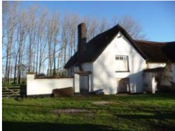
North west gable and wall towards linhay
