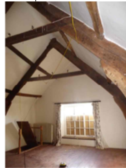
Bedroom 1 with exposed trusses
