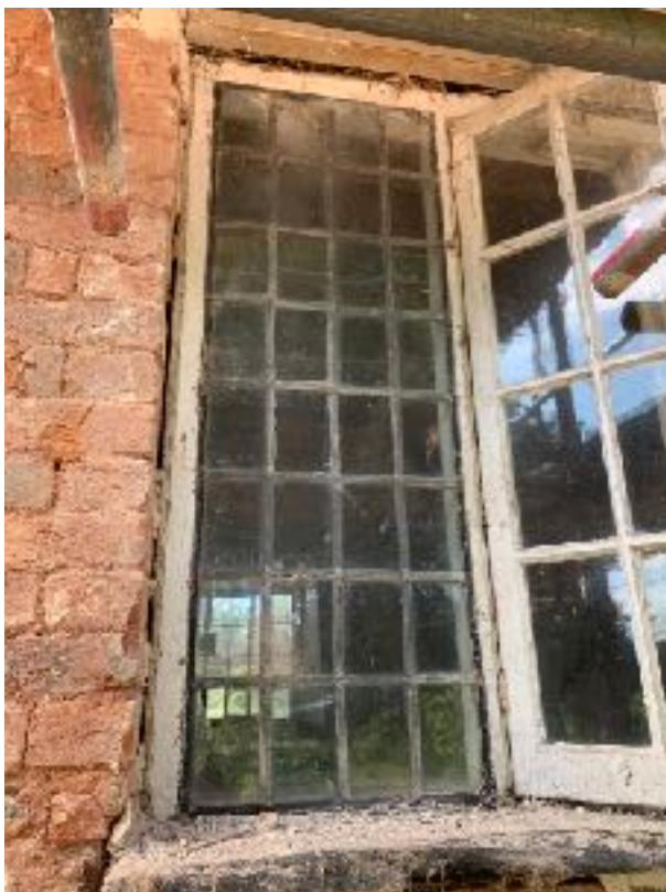
Previously: Cast cill inserted into window frame, causing rotting of frame. Bottom rail of soft wood frame has not
