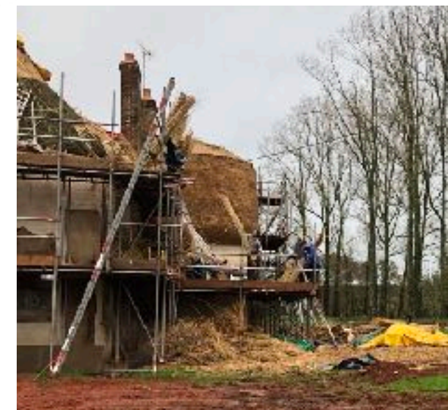
Side view of outshut from south. Thatching work in progress December 2020
