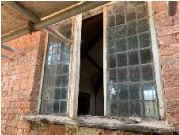
Previously: Cast cill inserted into window frame, causing rotting of frame. Bottom rail of soft wood frame has not
