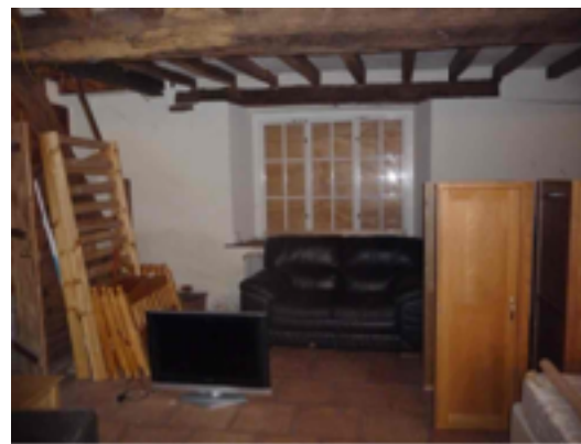
Kitchen south east end with stair to first floor corner
