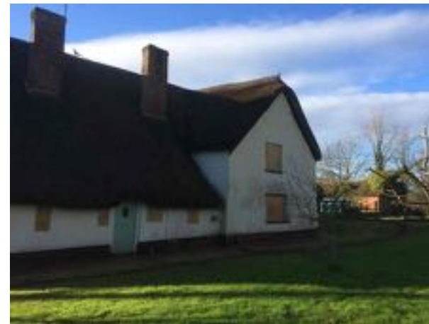
North eastern elevation of Farmhouse
