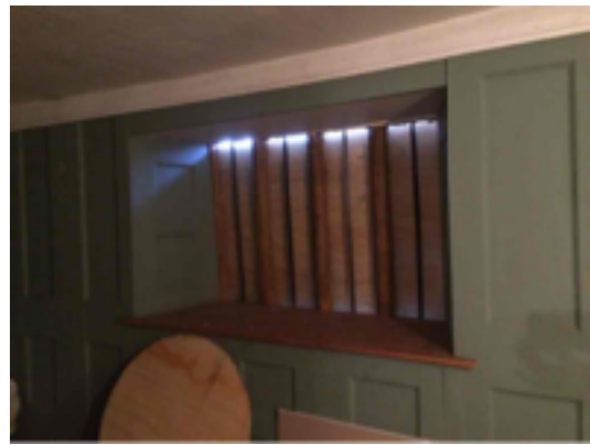
'North' 17C window in 20C panelling to Dining Room
