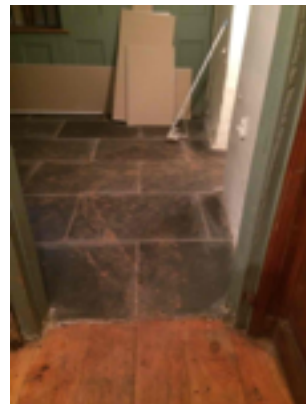
Transition of floor finishes Drawing Room to Dining Room
