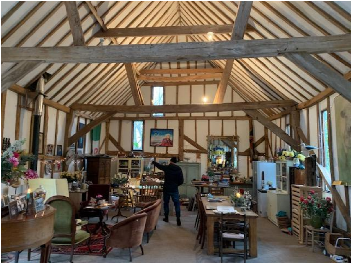
Figure 7: Highbuilding Farm barn interior
