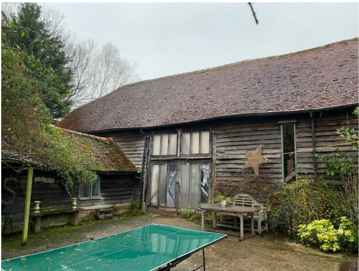
Figure 6: Highbuilding Farm barn, south side
