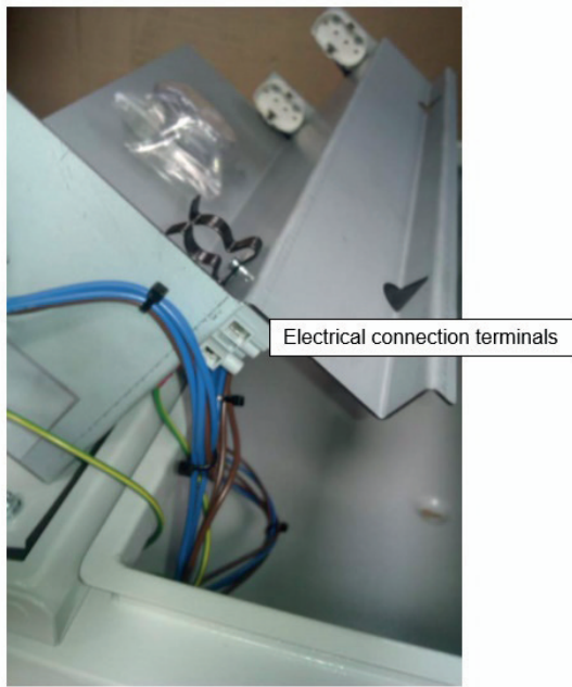
Figure 23 - Electrical Connections
