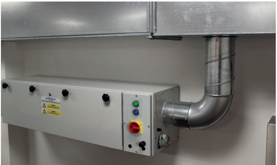
Figure 6 - UV-O 1000 Unit Installed
