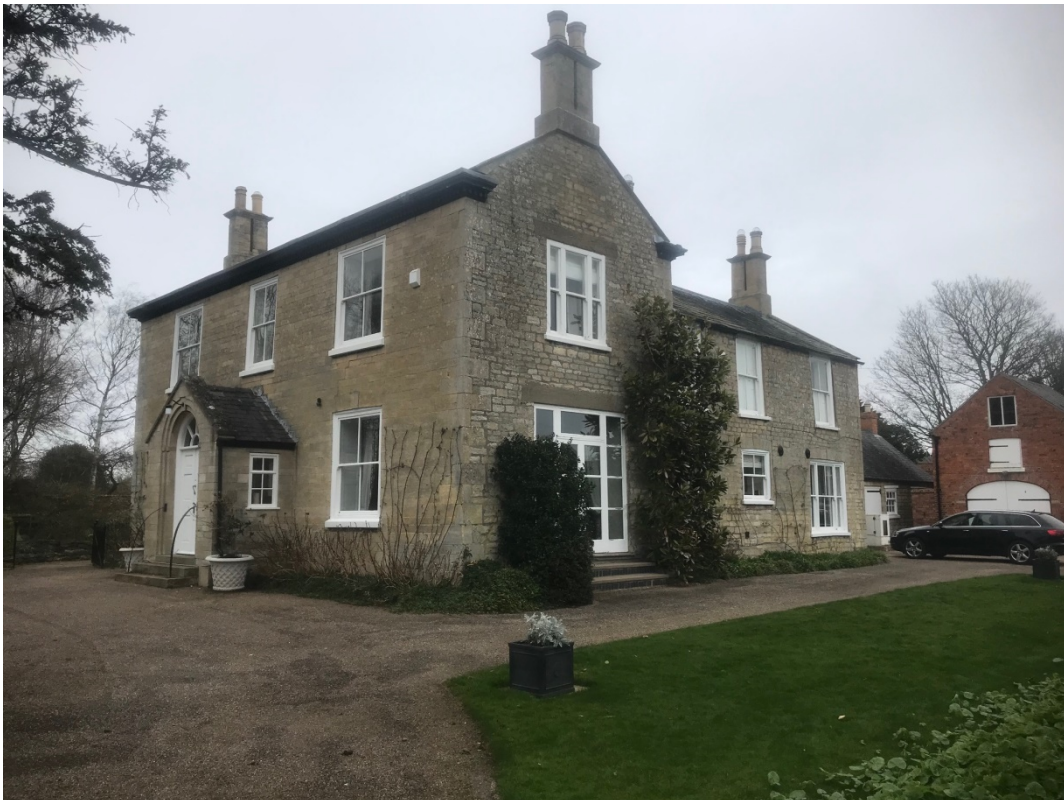
(Osbournby House – South & West elevations)
