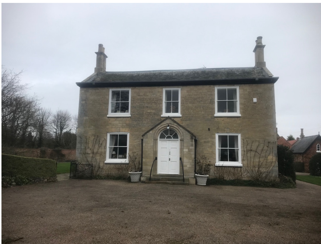
(Photograph of West Elevation 5 x main windows)
