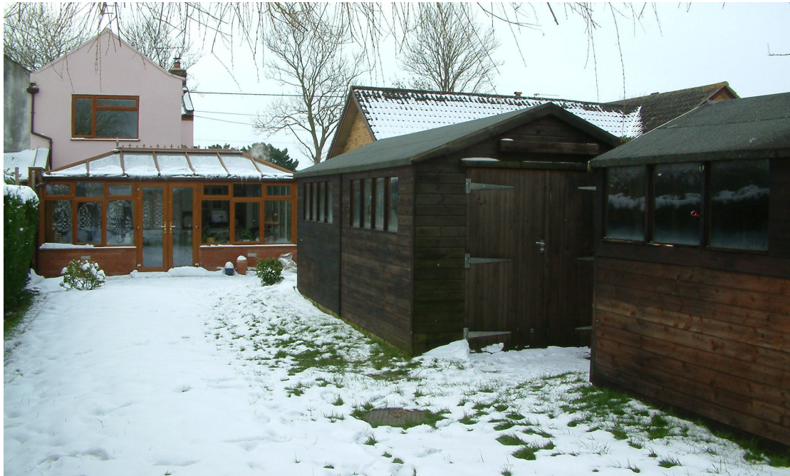
Photograph 3: Photograph of existing outbuildings taken from the north
