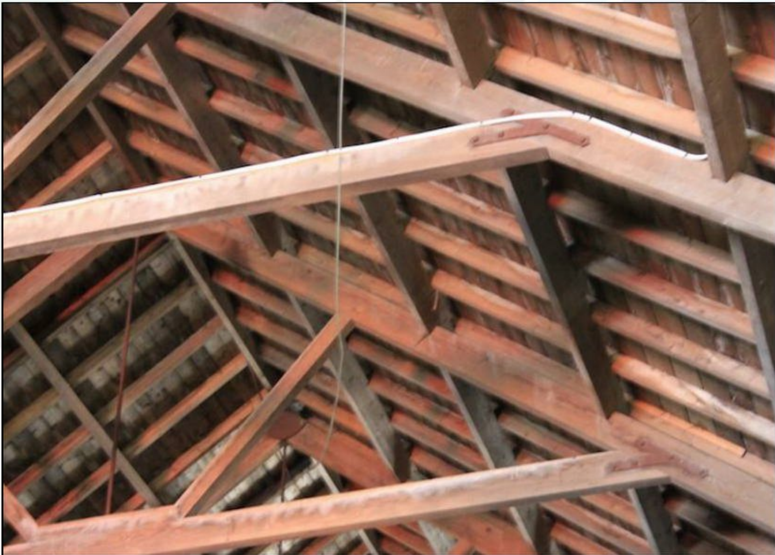
Figure 8. Slates laid onto wooden sarking and joists.
