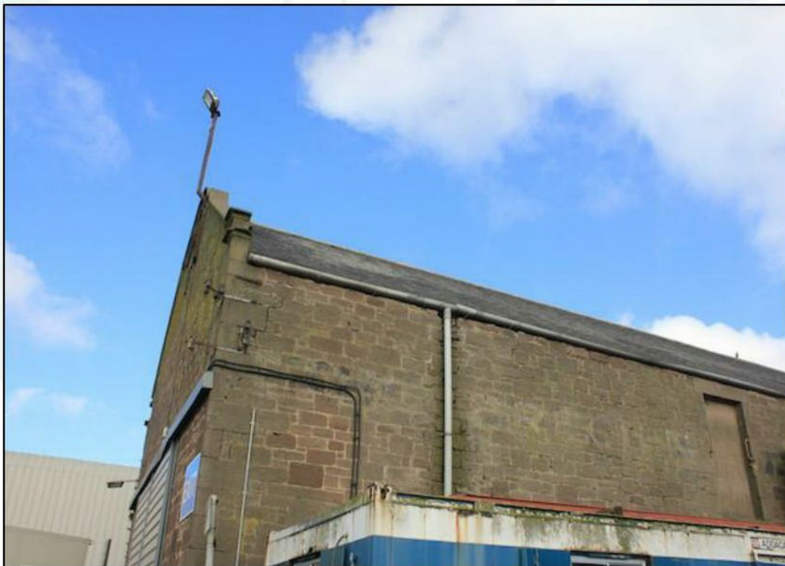
Figure 2. Stonework construction of warehouse.
