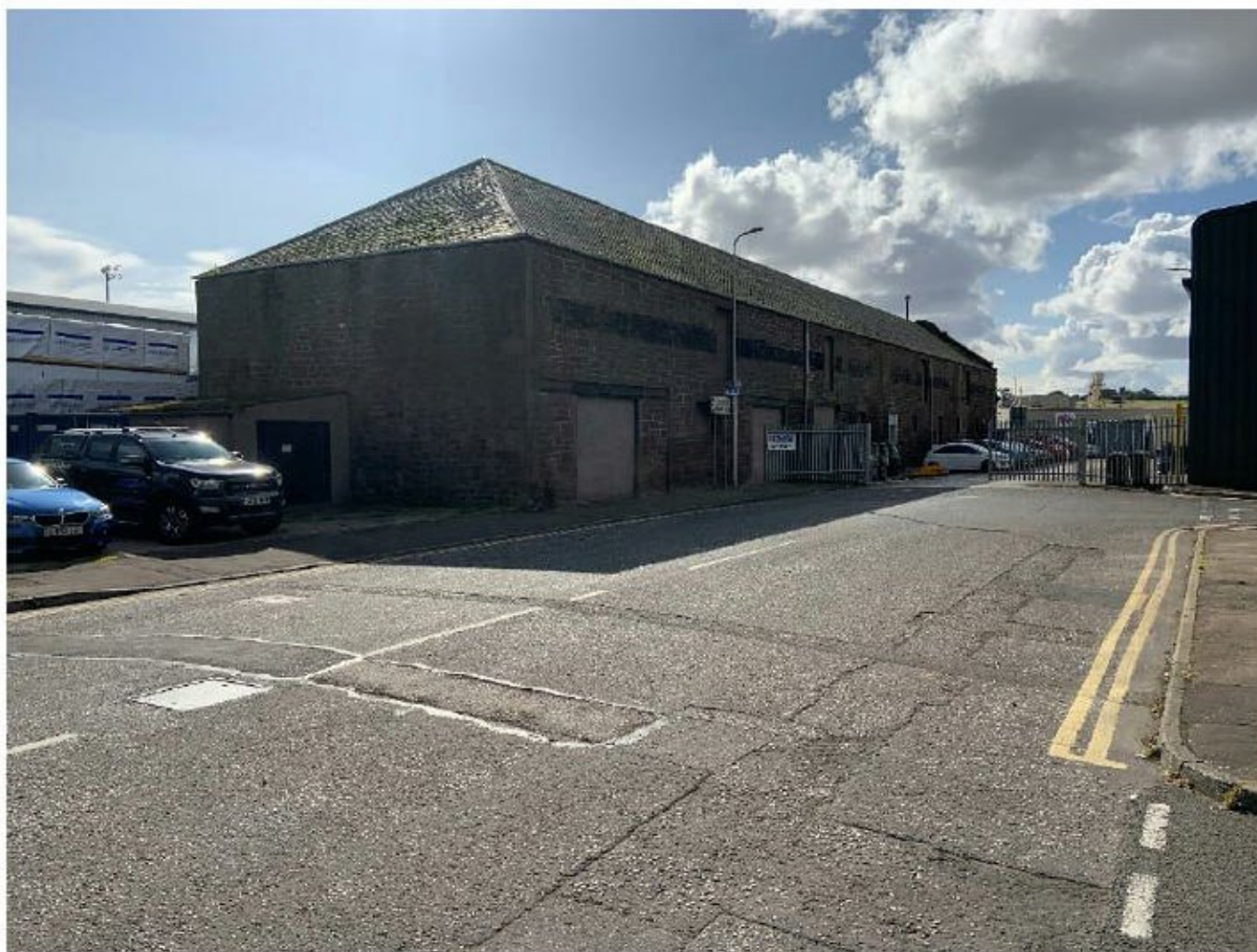
Figure 2: North East Gable & North West Elevation (Meridian Street)
