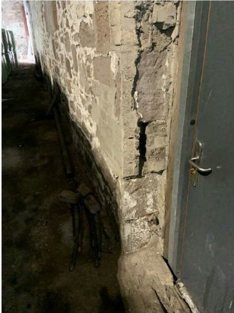
Figure 25: Damaged Stonework
