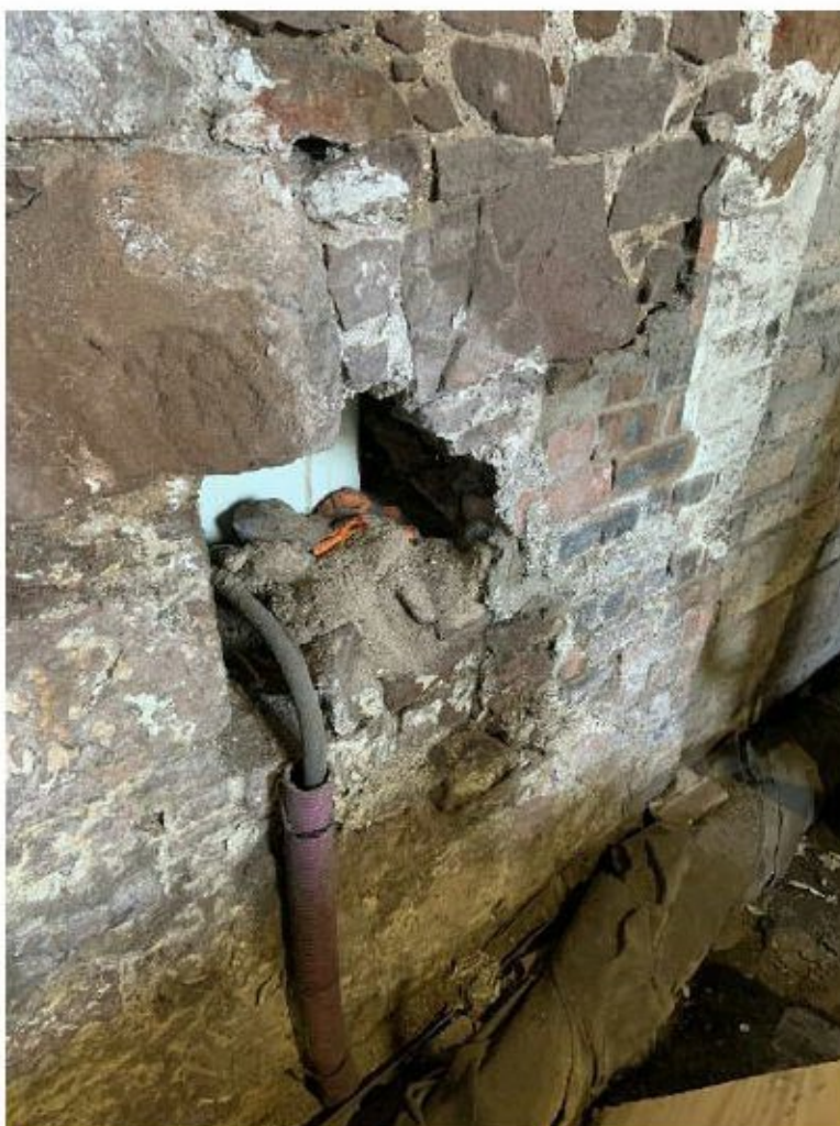
Figure 24: Damaged Stonework
