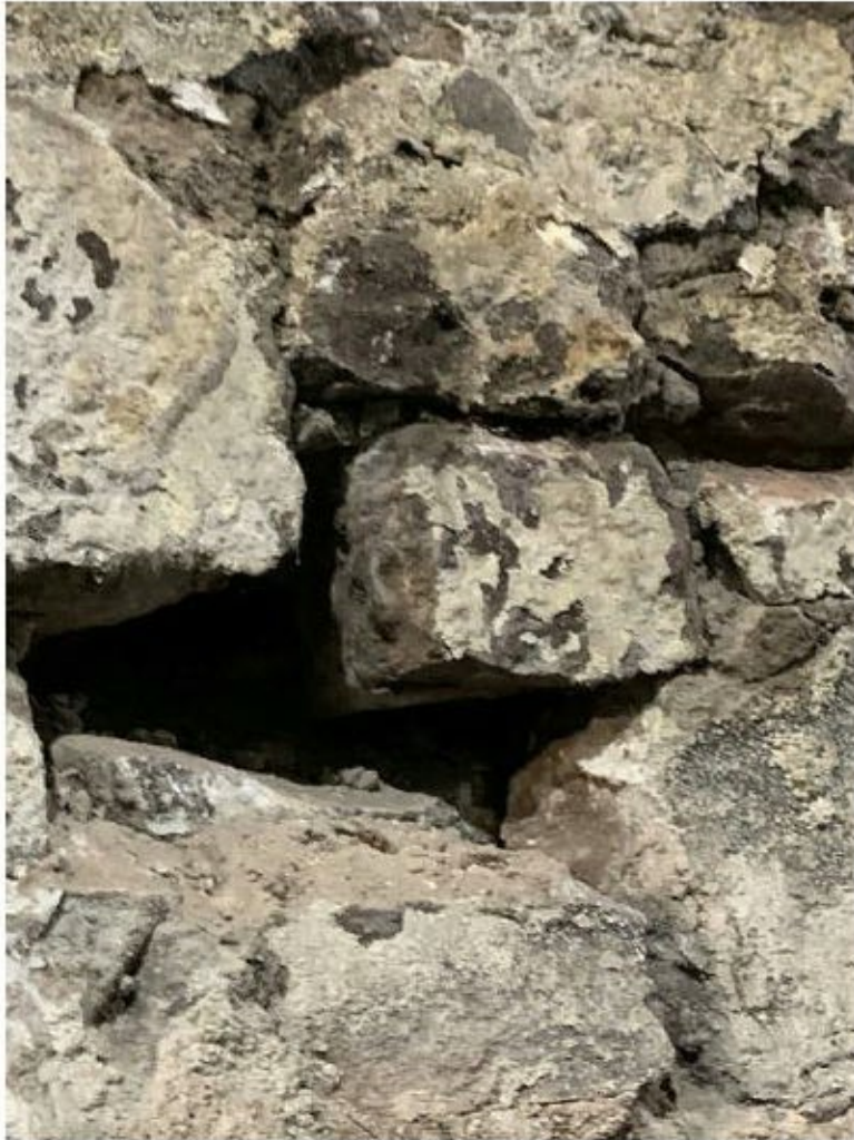
Figure 29: Damaged Stonework
