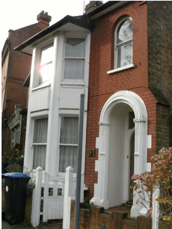
Front garden wall and picket gate
