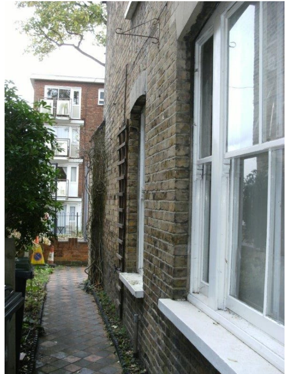
Existing path to side access
