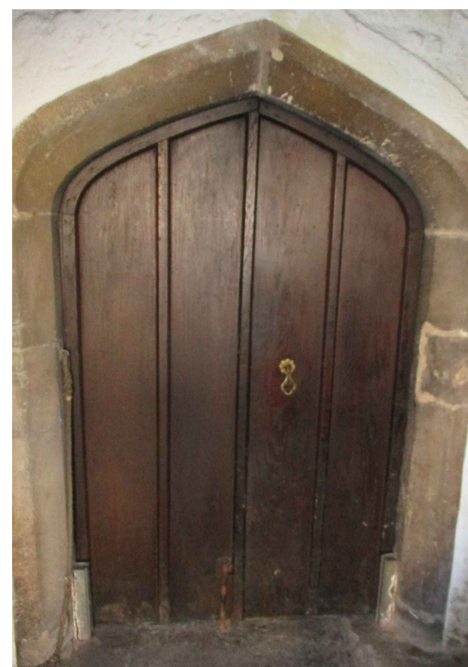
Existing Photo 1 North Porch Lobby Door Viewed from the Porch
