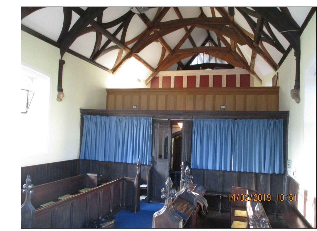
The Chapel interior looking west with the medieval curtain covered screen in front and the modern timber balustrade behind. A further modern screen at gallery level further sub-divides the original space.
