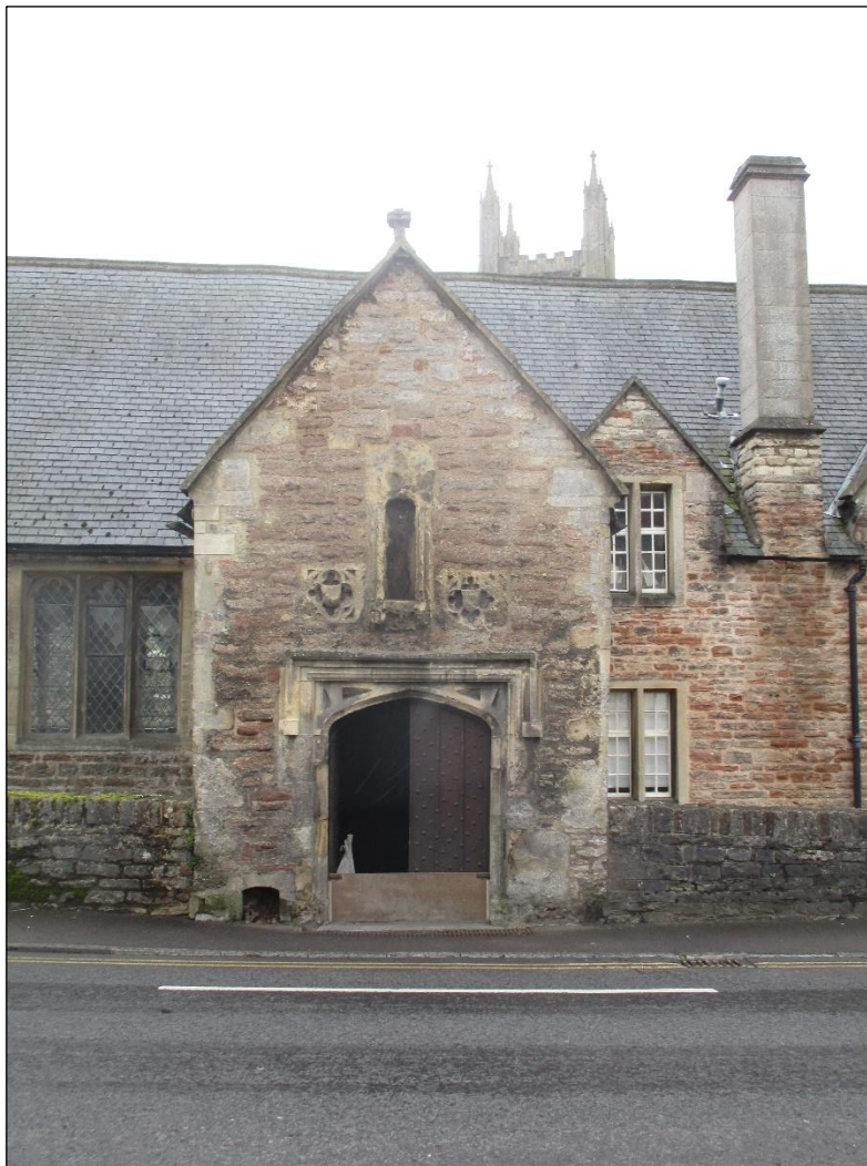
Above: The north porch.
