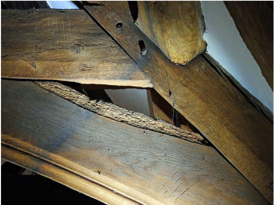
Carpenters' assembly marks: Truss 4, west face, north and south with differencing.
