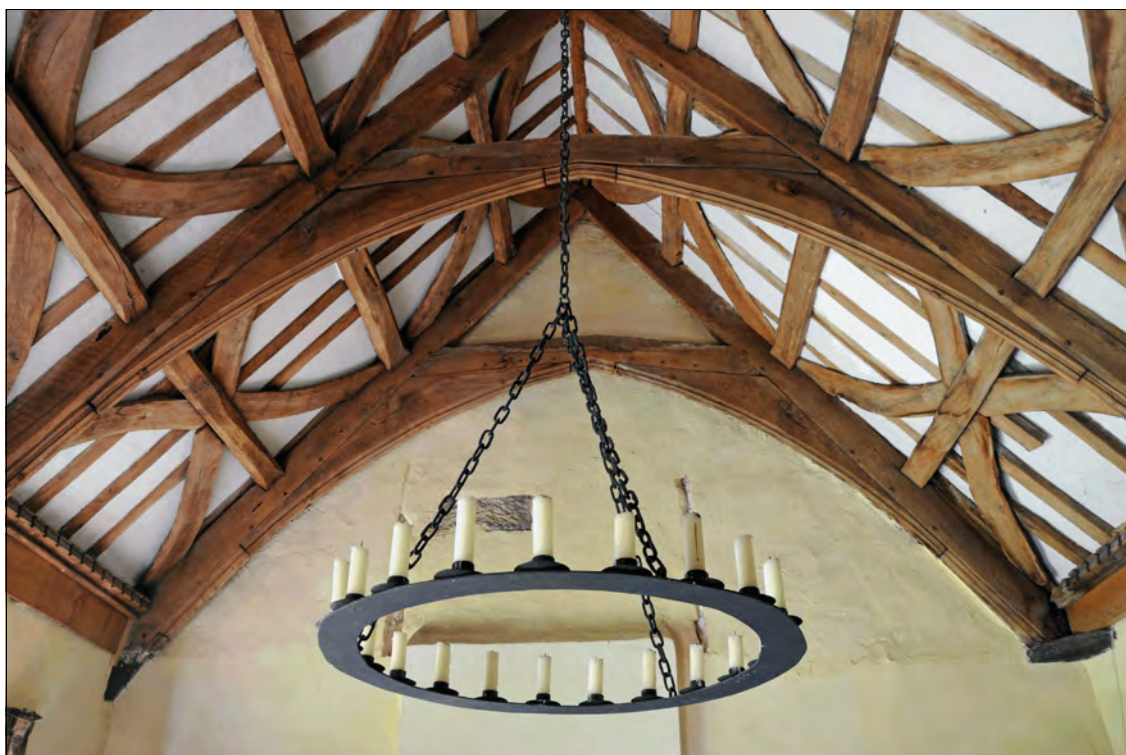
The fifteenth century hall roof looking east (top) and west (below)
