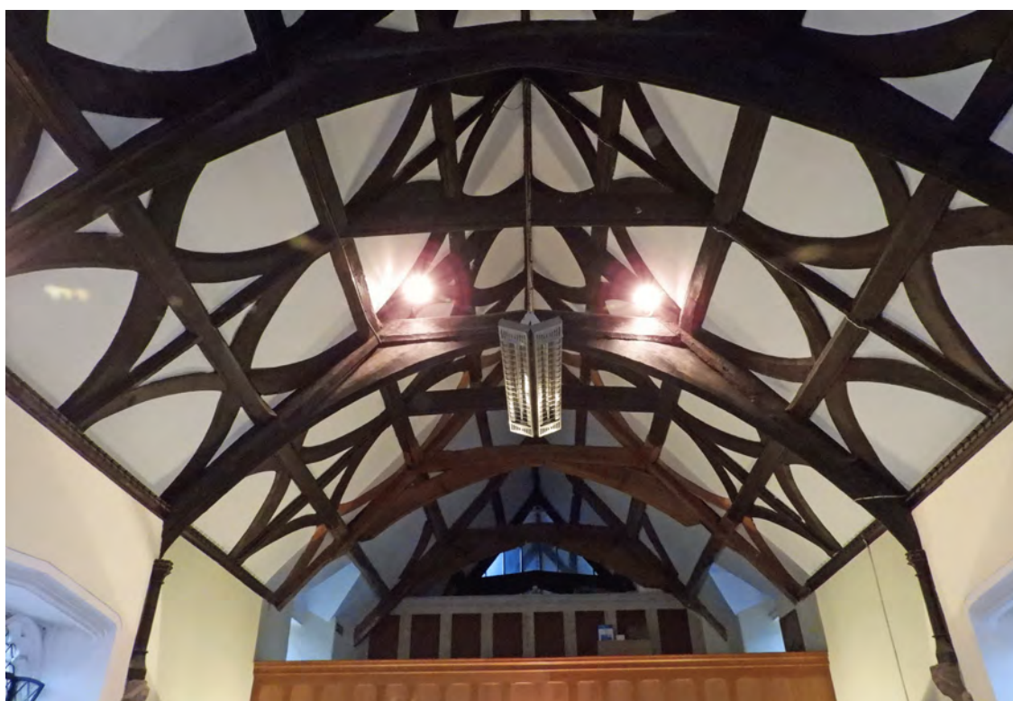
The Chapel roof looking east (top) and west
