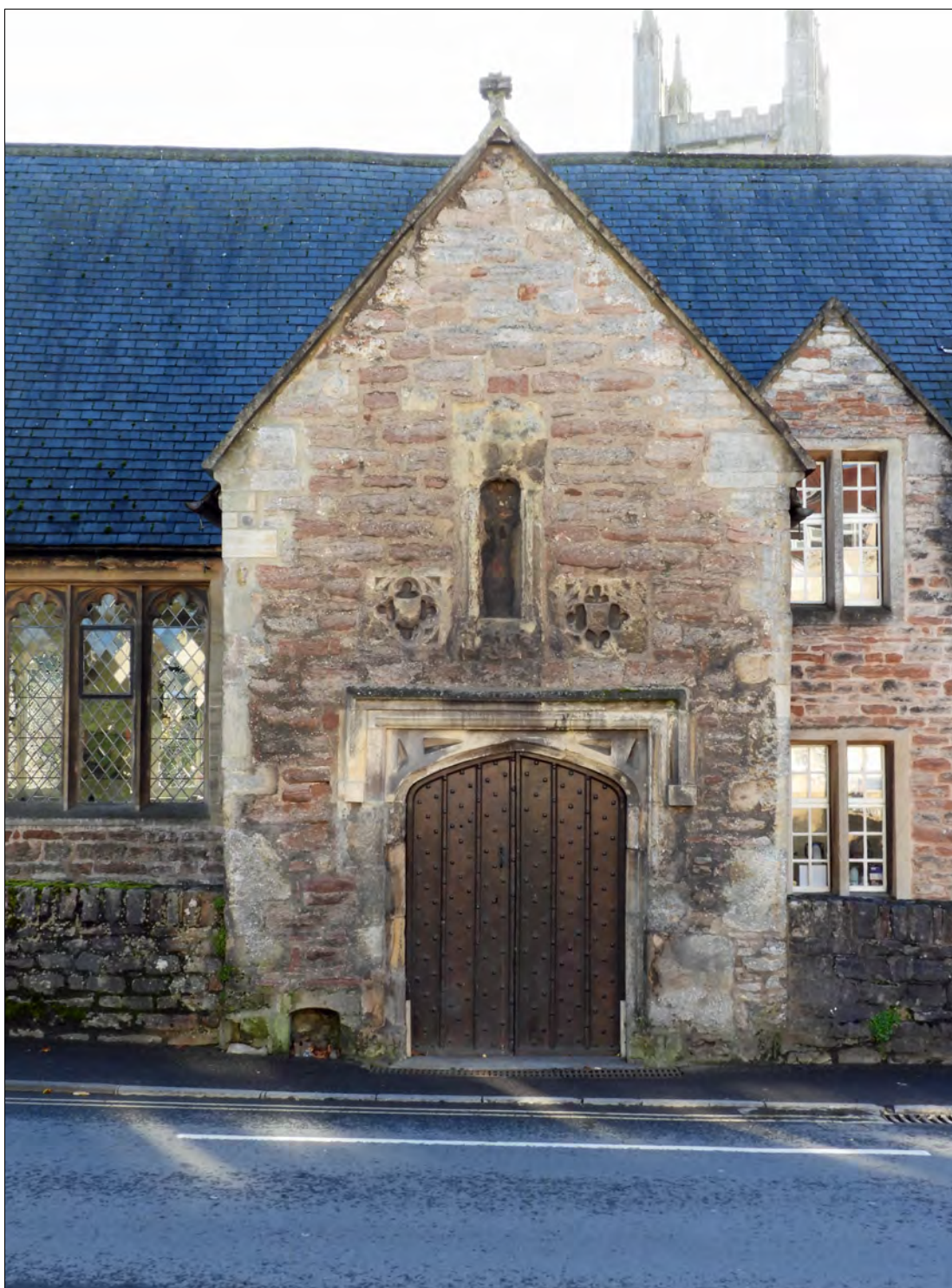
The north elevation of the north porch
