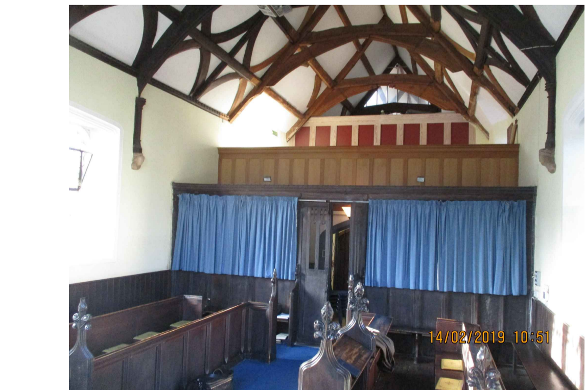
The Chapel interior looking west with the medieval curtain covered screen in front and the modern timber balustrade behind. A further modern screen at gallery level further sub-divides the original space.
