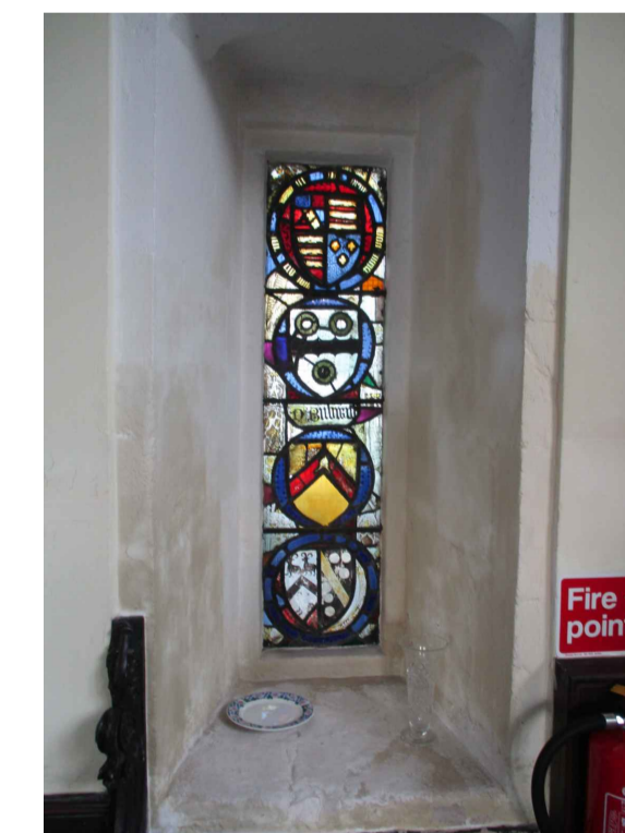
The medieval glass in window NIII. The window has been the subject to a specialist conservation report prepared by Holywell Glass.
