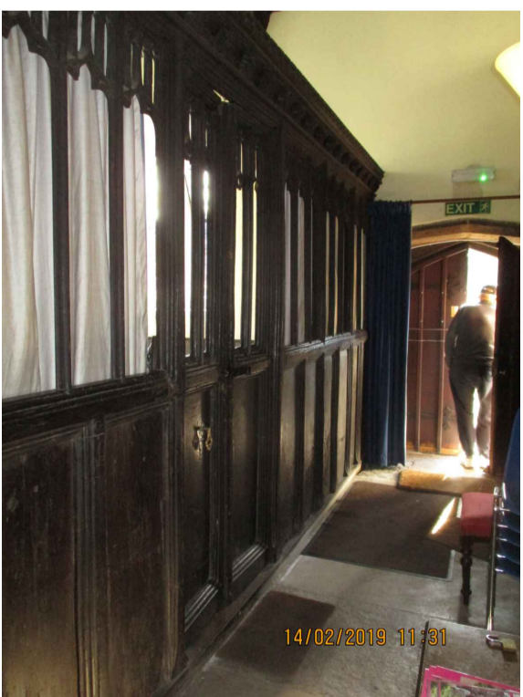
The passage with medieval screen. The floor is a combination of stone and concrete.
